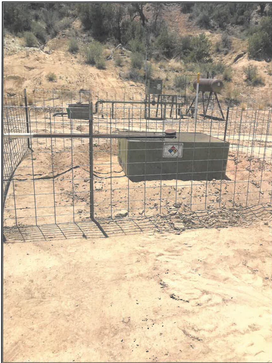
PHOTO 3: AST Taking Place of Closed BGT
