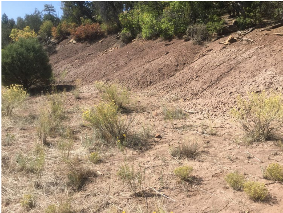
Well Pad Cut Slope, Showing some Erosion
