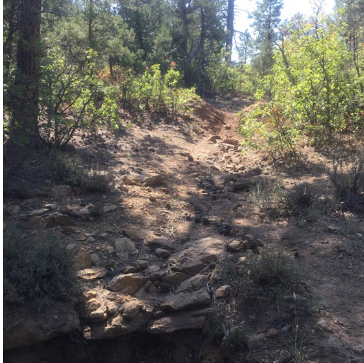
Erosion along Access Road
