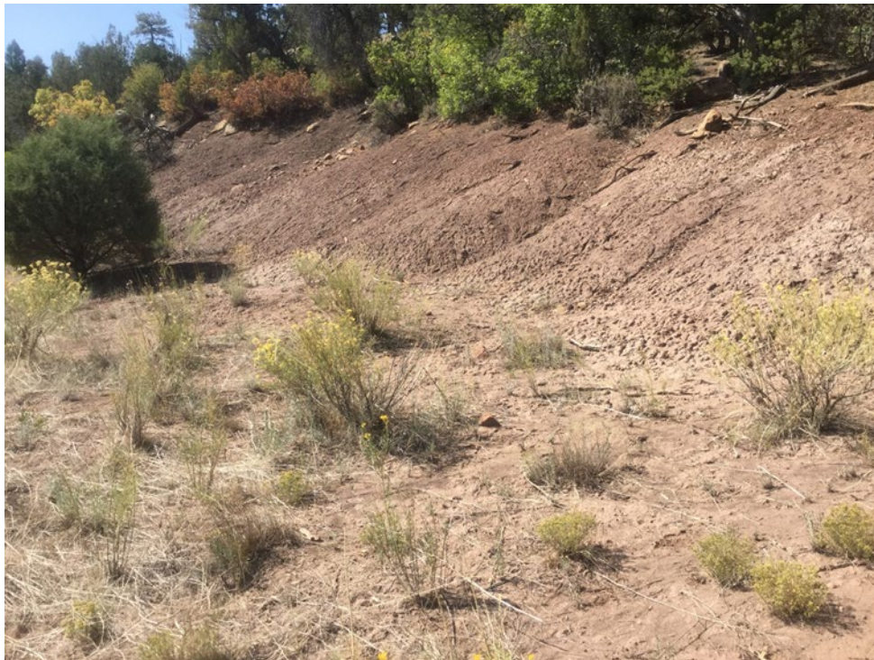
Well Pad Cut Slope, Showing some Erosion
