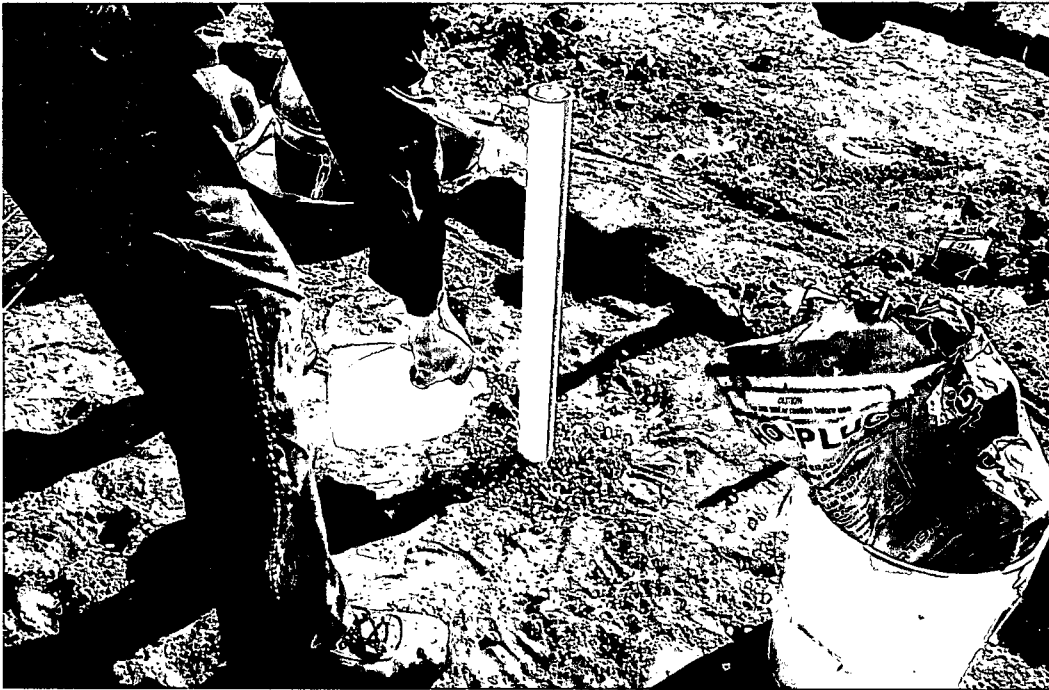
Photo 3: View of the soil vapor extraction well.
