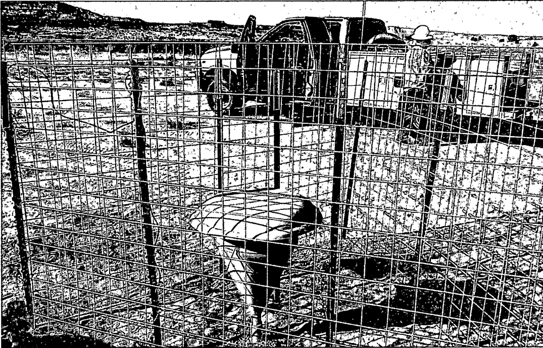
Photo 5: View of the soil vapor extraction ventilation system with security fencing.
