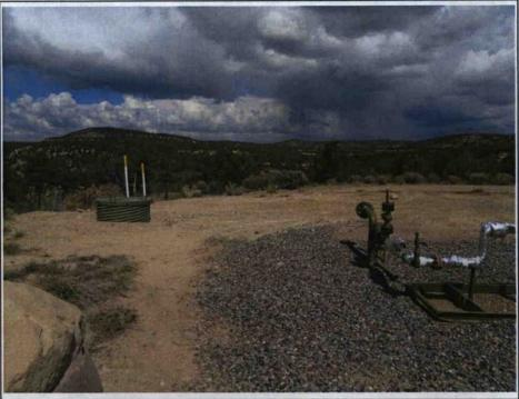
Description: Facing NW, looking at former BGT location. Area has been backfilled with clean fill dirt and compacted.
