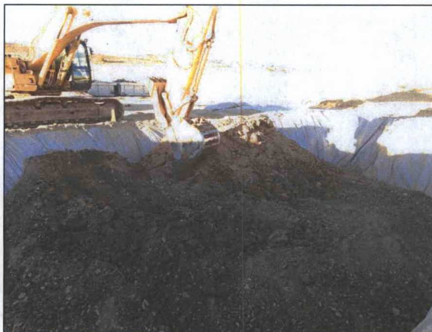
Figure 4: Spreading the mixed cuttings in the burial trench.
