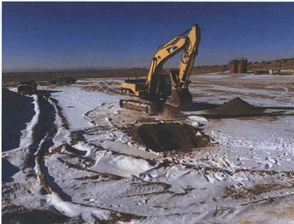
Figure 1: Excavating the cuttings trench.
