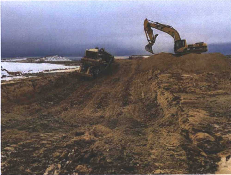
Figure 1: Excavating the cuttings trench.
