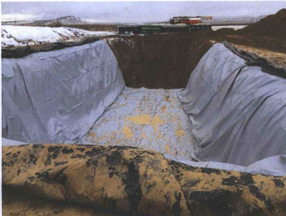
Figure 2: Lining the cuttings trench.
