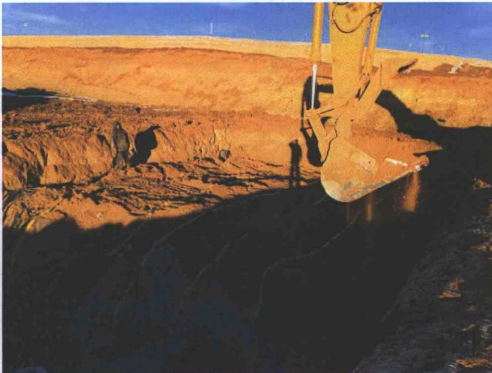
Figure 4: Placing clean soil on top of lined mixed and stabilized drill cuttings. Caution tape marks the top of the liner cap.
