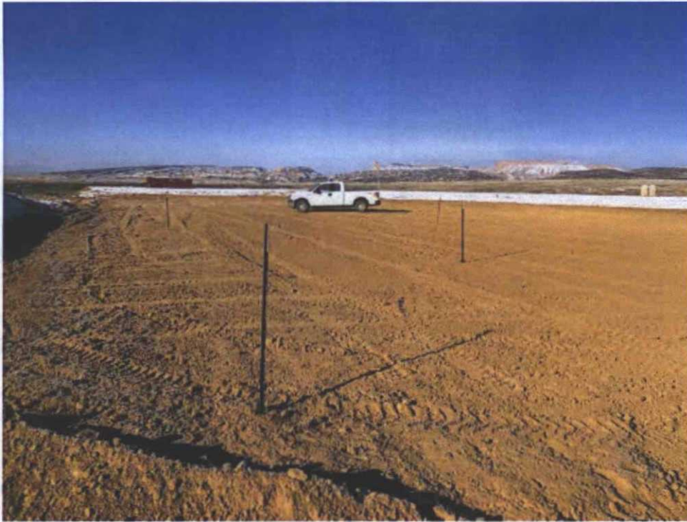
Figure 5: Final cuttings trench grade with T-posts marking cutting trench corners and center.
