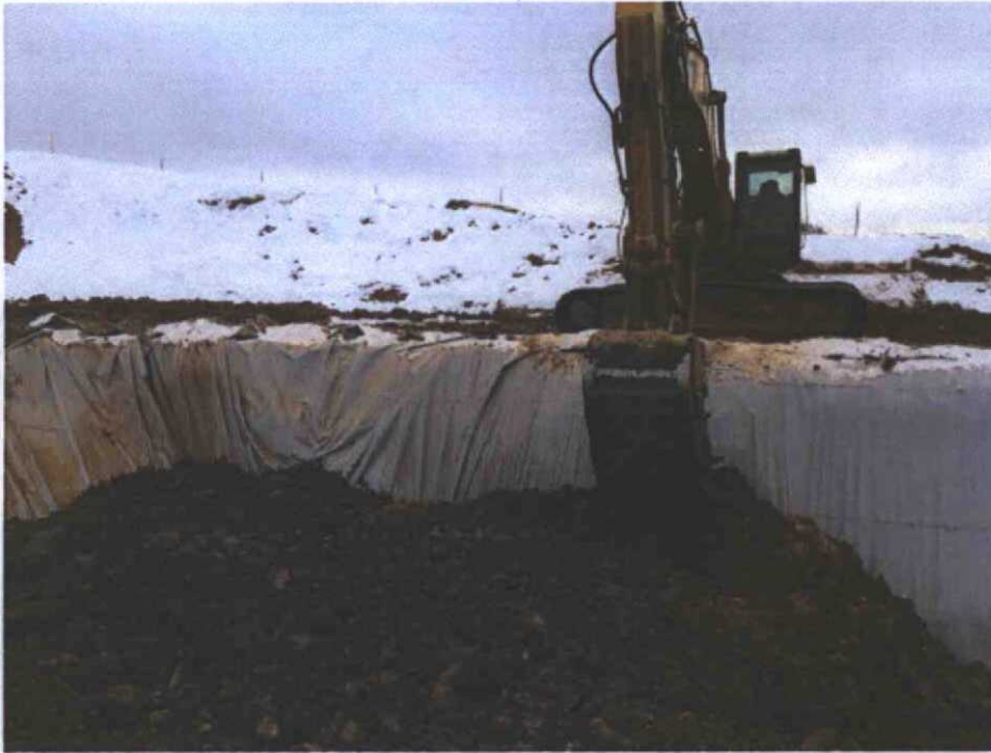
Figure 3: Mixing clean soil with drill cuttings.
