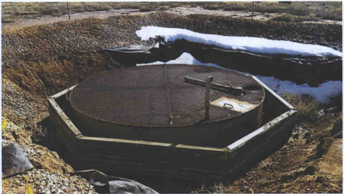
Photograph 1. General view of below grade tank in place before closure activities.
