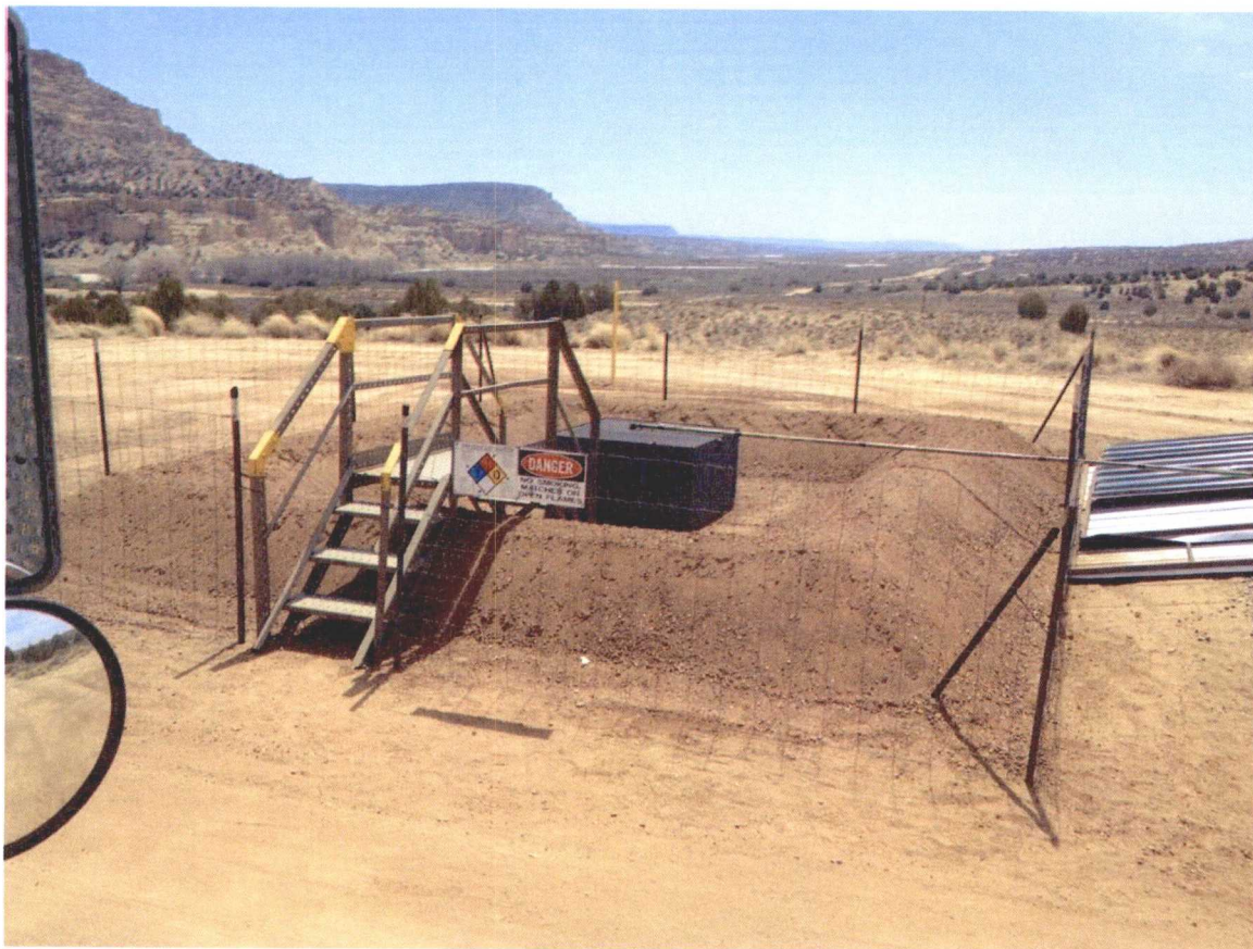
PHOTO 1: BGT Area after set of new Above Grade Tank
