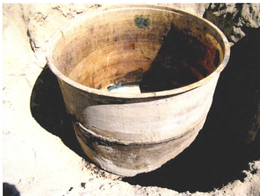
Photo 2: Subject below grade tank with visibly stained soil at the base of the tank pit.
