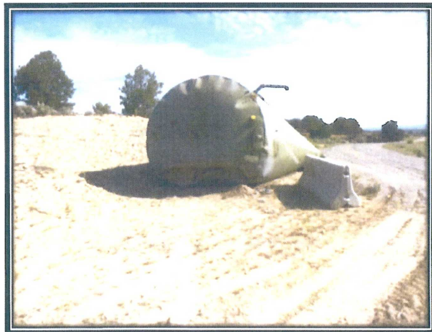
Picture 2: View of Tank Struck by Lightning
