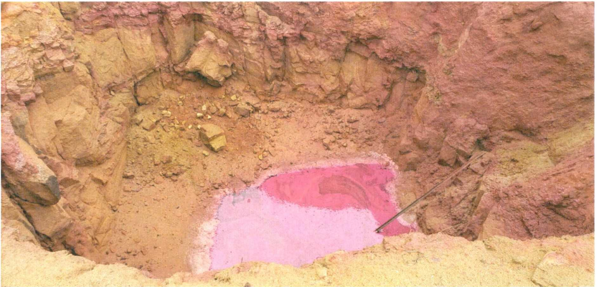
Photo 4: Excavation upon application of potassium permanganate. Photo taken October 24, 2018.
