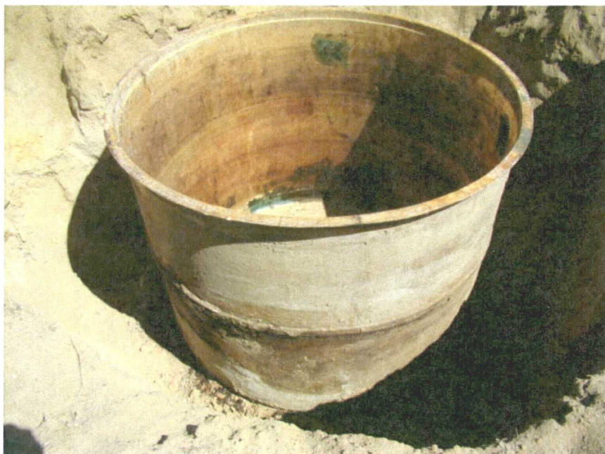
Photo 2: Subject below grade tank with visibly stained soil at the base of the tank pit. Photo taken August 29, 2018.
