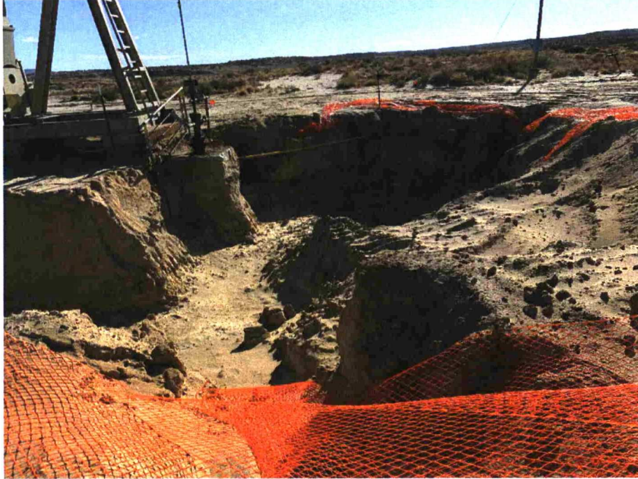
Photo 1: West excavation adjacent to pump jack. Date taken: 11/5/2018.
