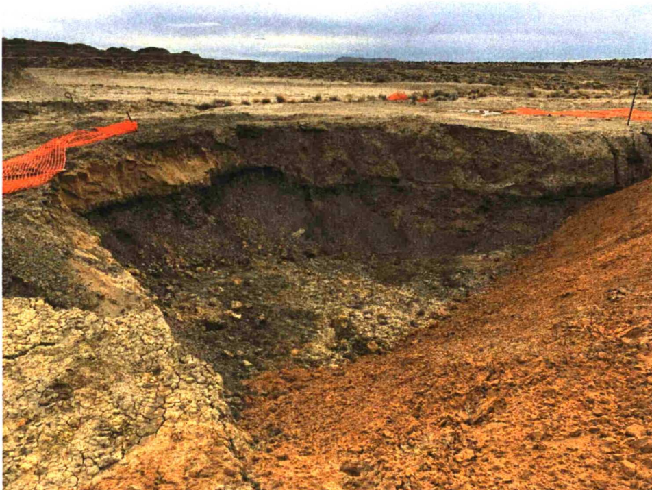
Photo 6: East excavation after initial backfill and SC-27 through SC-29 sampling and prior to final backfill. Date taken: 3/11/2019.
