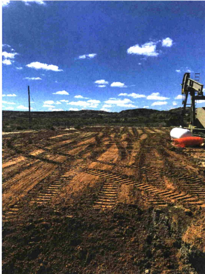
Photo 7: Final backfill of east excavation. Date taken: 3/15/2019.
