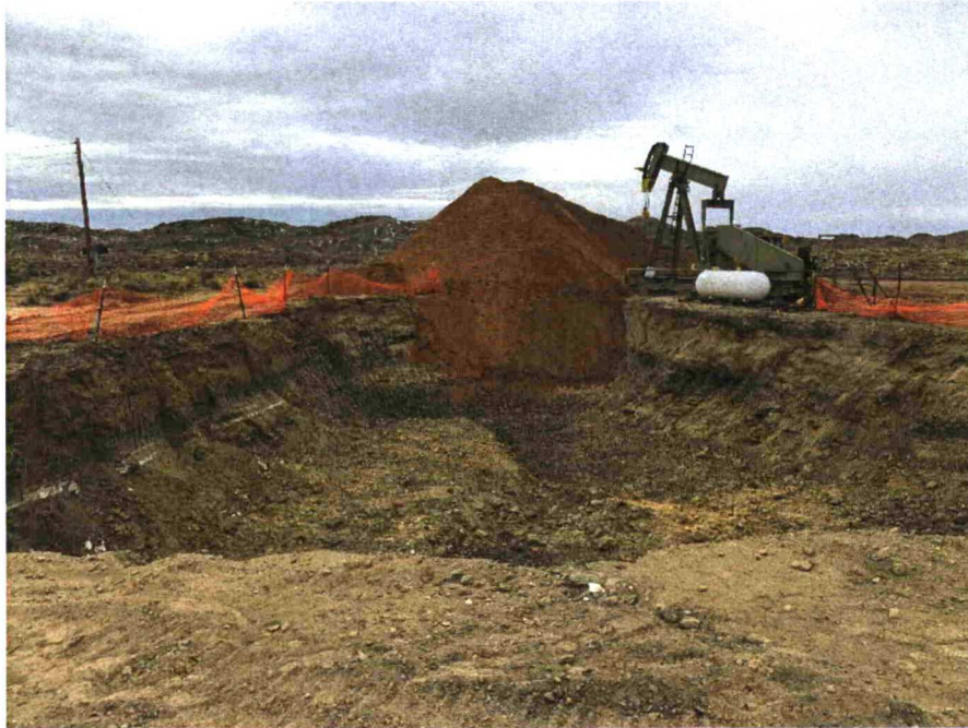
Photo 3: East excavation prior to initial backfill and SC-27 through SC-29 sampling. Date taken: 2/14/2019.
