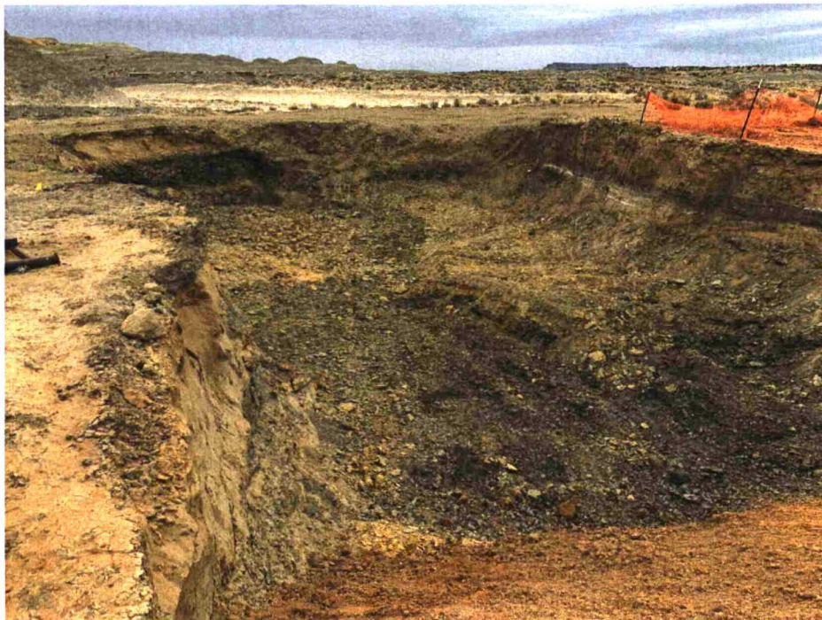
Photo 4: East excavation prior to initial backfill and SC-27 through SC-29 sampling. Date taken: 2/14/2019.
