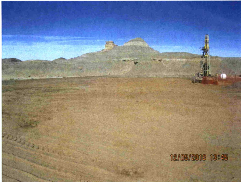
Photo 5: Final backfill of west excavation. Date taken: 12/5/2018.
