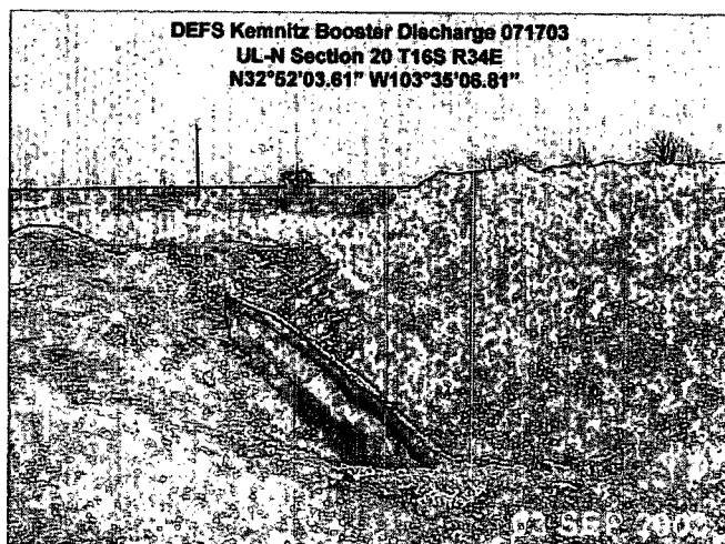
Site ready for pipe section replacement; stockpiled topsoil on east side of pipeline
