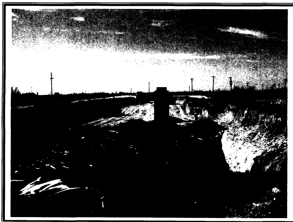
Installation of plastic liner in associated pit at north end of tank battery excavation
