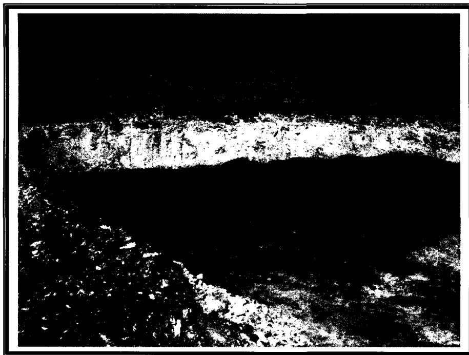
Clay liner inside associated pit excavation
