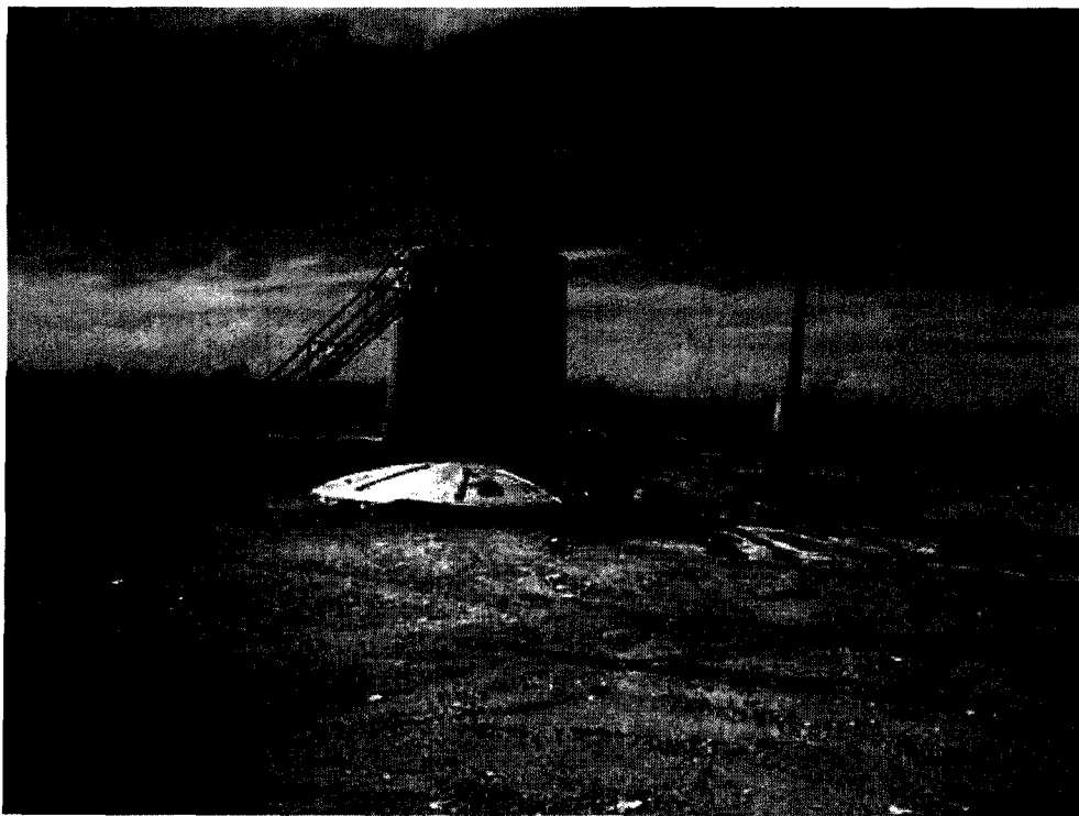
Photograph #2- Looking westerly at fiberglass tank with top in foreground. Fluid and dark stained soil indicate contamination.
