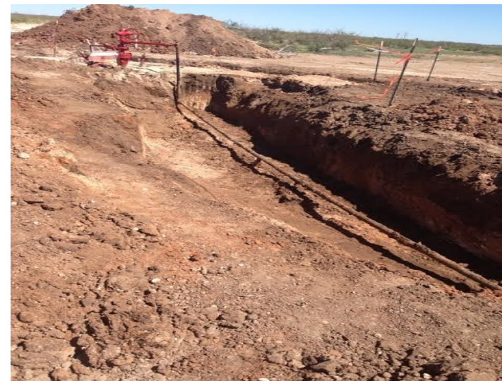
Excavation of injection line 10-14-14
