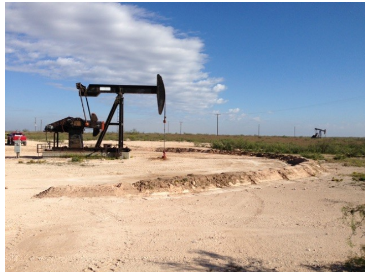
Pad at completion of firewall 10-17-14
