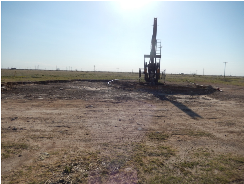
Excavation South of Well Viewing West, April 21, 2015
