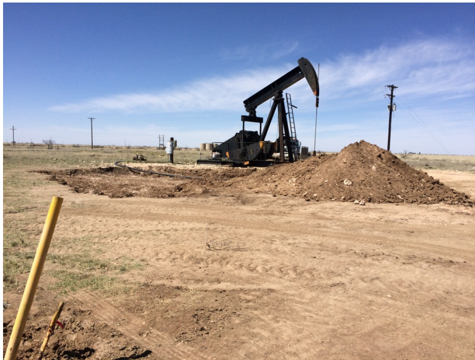
Excavation South of Well Viewing North, April 7, 2015
