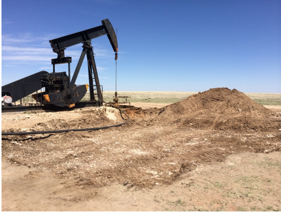
Excavation South of Well Viewing Northeast, April 7, 2015
