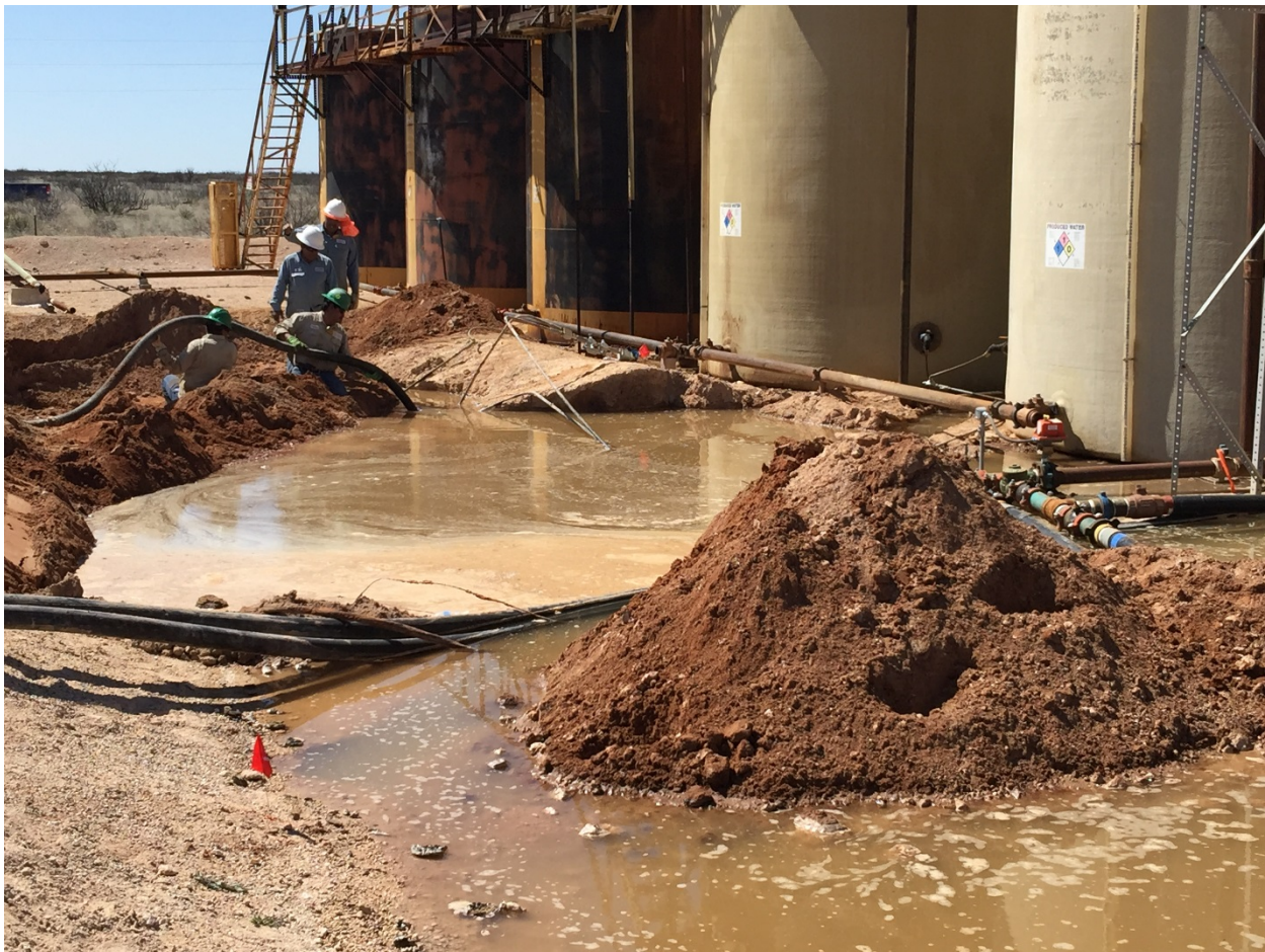
Second spill inside bermed area. Fluid being recovered by vacuum truck
