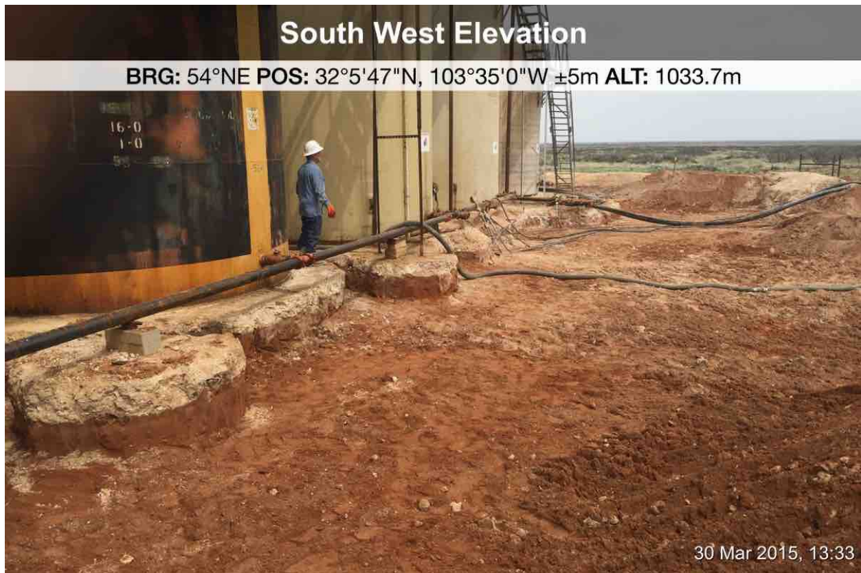
Spill area excavated to 2' bgs
