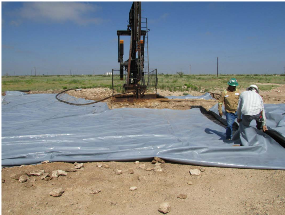
Installing Liner in Excavation Viewing West, June 22, 2015
