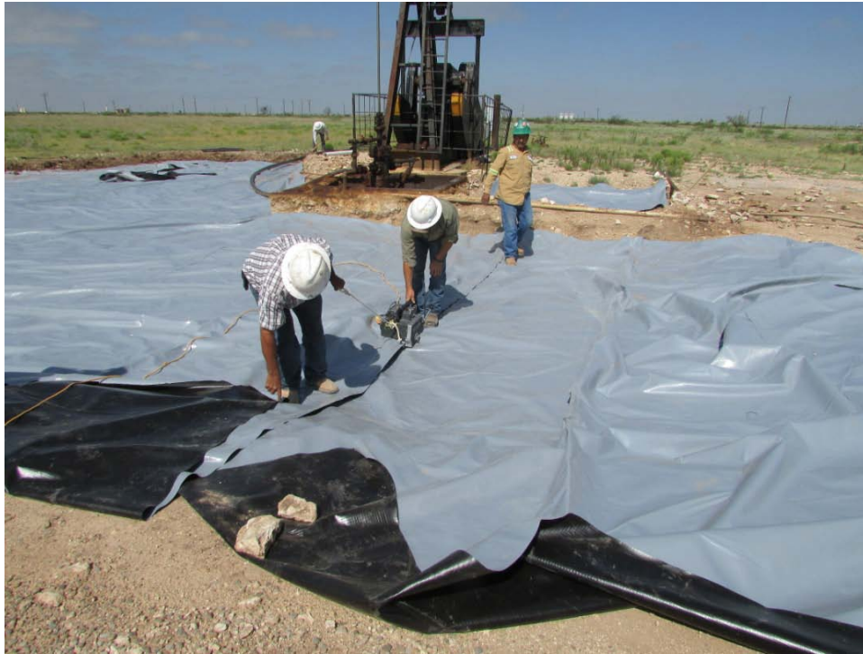
Welding Liner Seam, June 22, 2015
