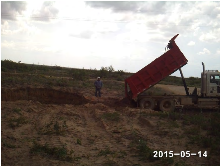
Importing soil to backfill north excavation, facing west
