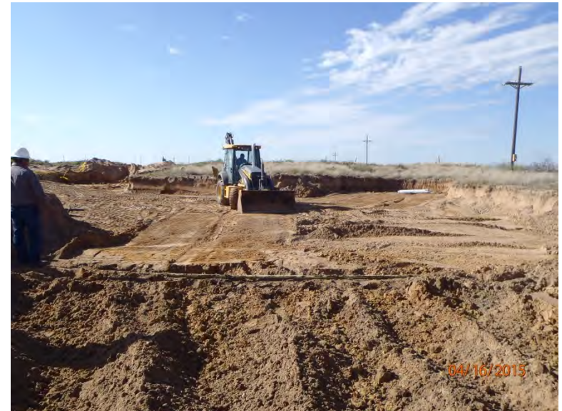
Leveling base of 4 ft excavation, facing south 4/16/15
