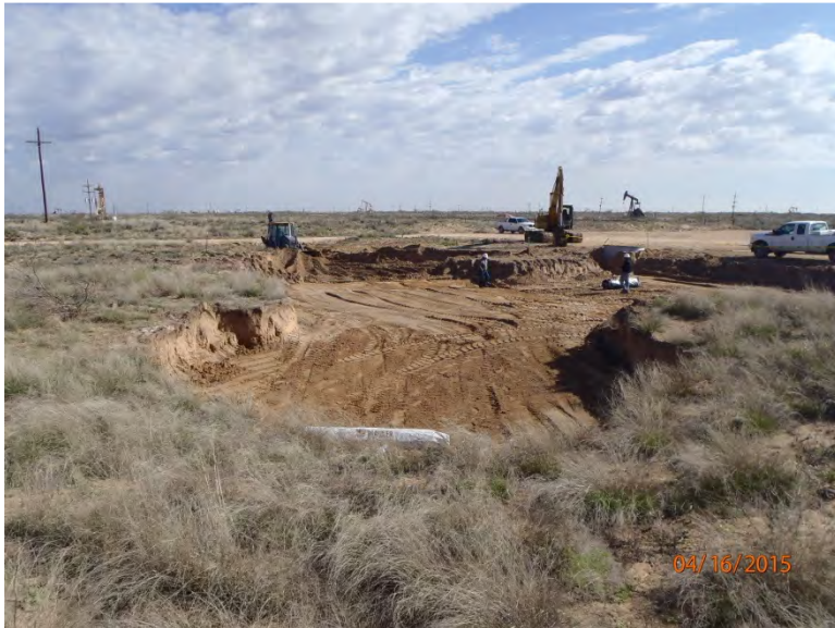
Excavation prior to liner installation, facing northeast 4/16/15
