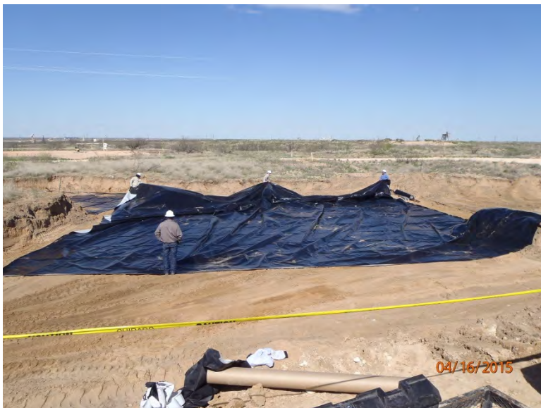
Installing liner, facing west 4/16/15
