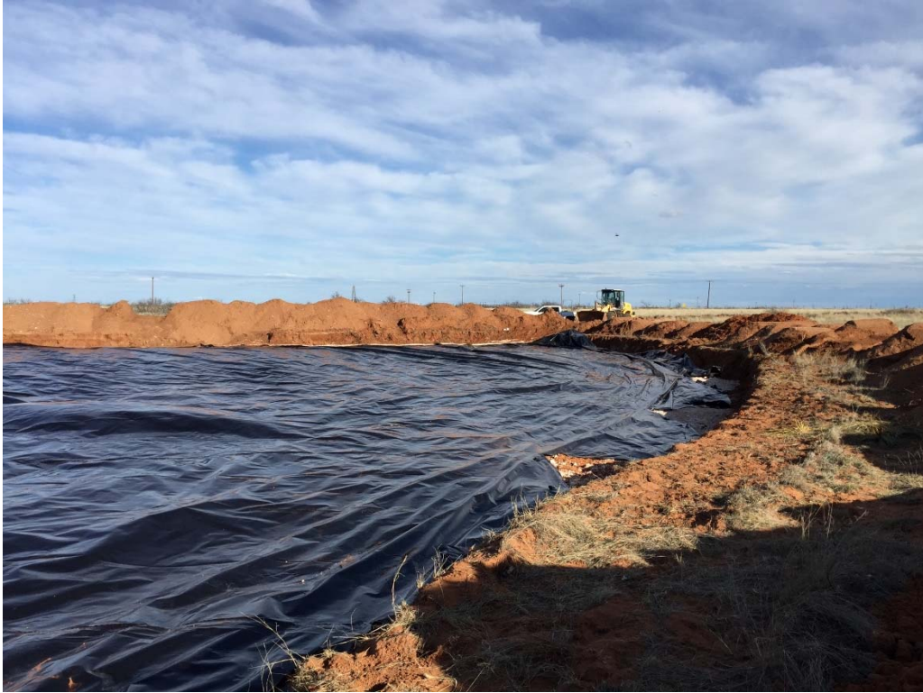
Photograph #3 – South liner installation
