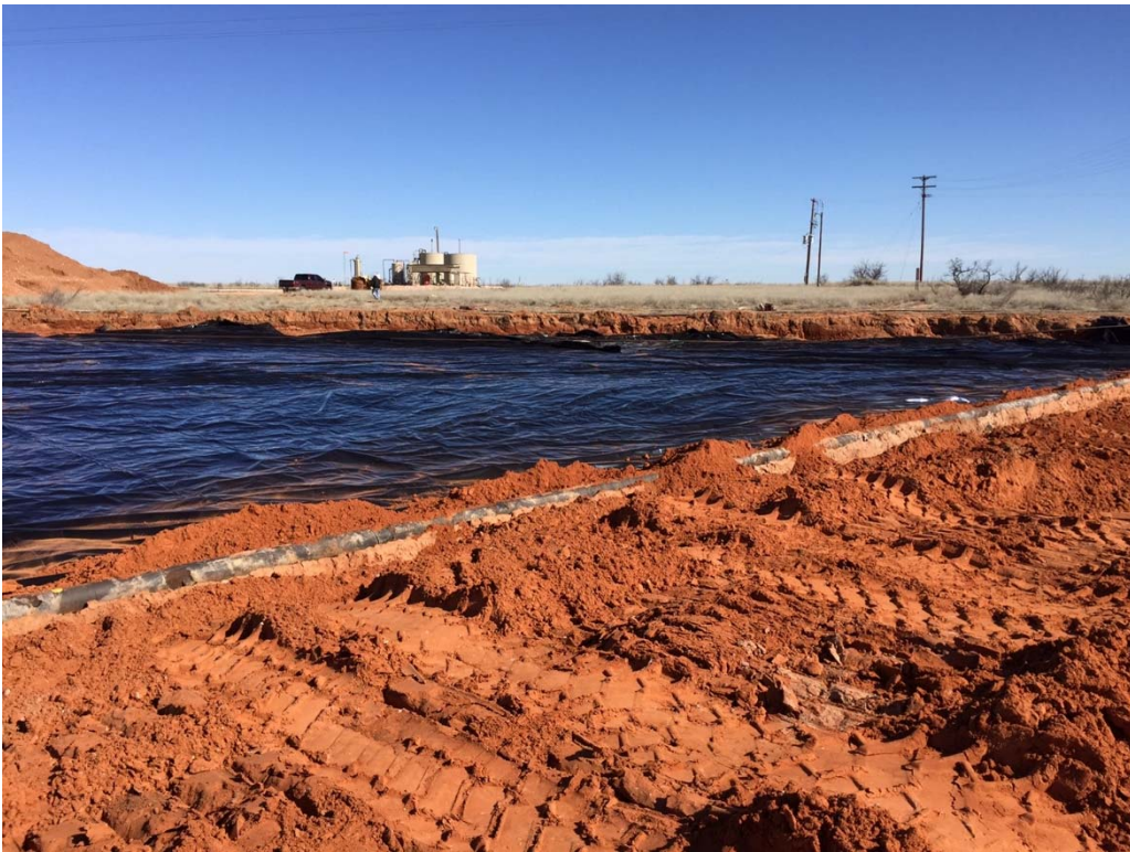
Photograph #6 – North liner installation
