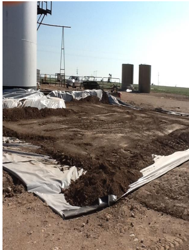
Liner Installation
