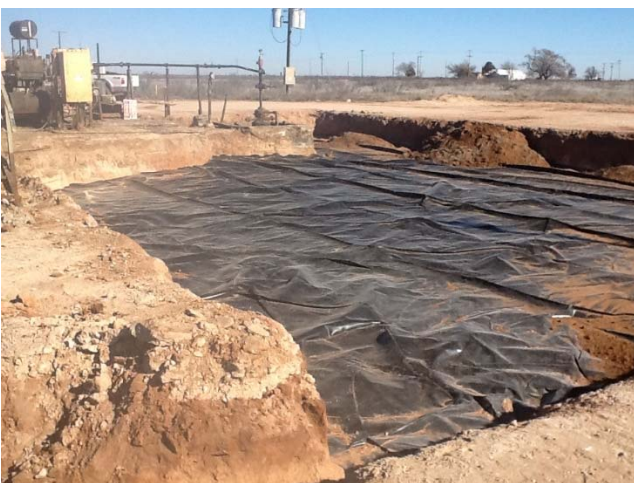
Lined north side layered topsoil
