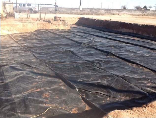
Lined Excavation facing north
