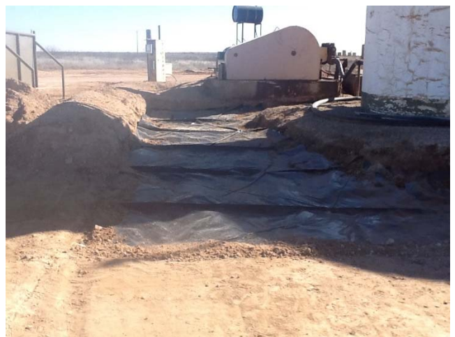
Excavated and lined west side of tanks
