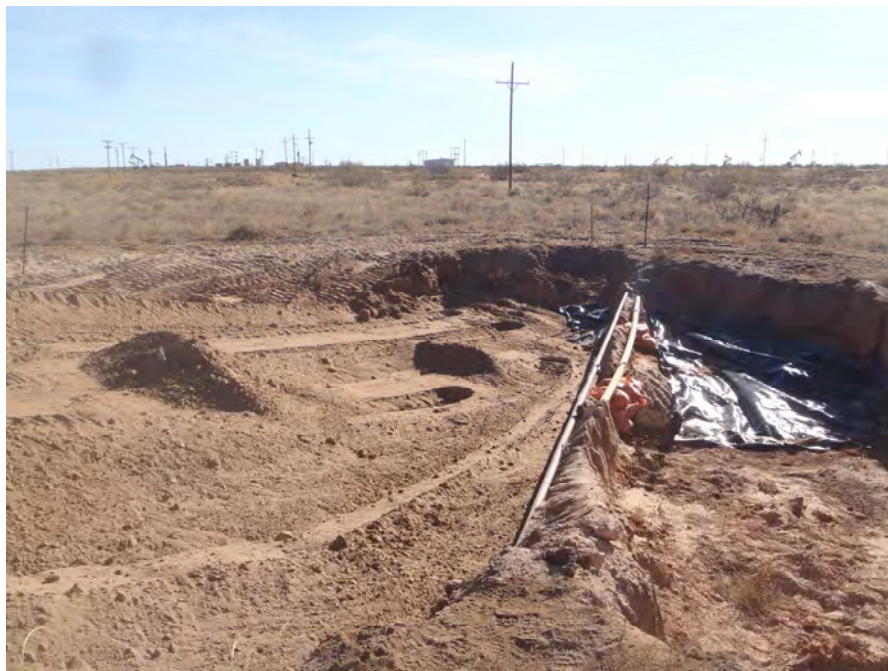
PHOTO 10: View of Supported Chaparral Water Injection Lines and Backfilling Activities - December 2012
