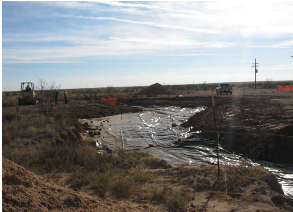
PHOTO 11: View of Backfilling Activities (20 mil Poly Liner) – December 2012
