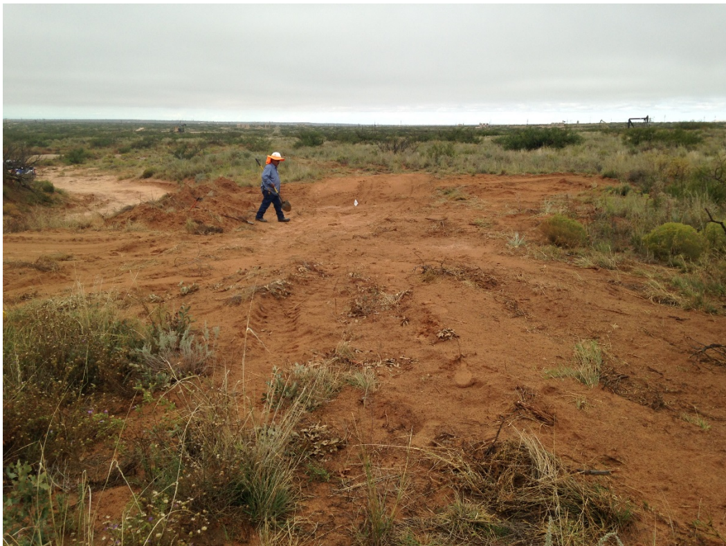
Spill area after initial scrape; collecting soil samples
