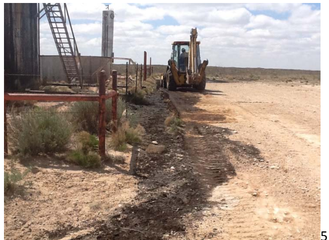
Surface Removal of north side
