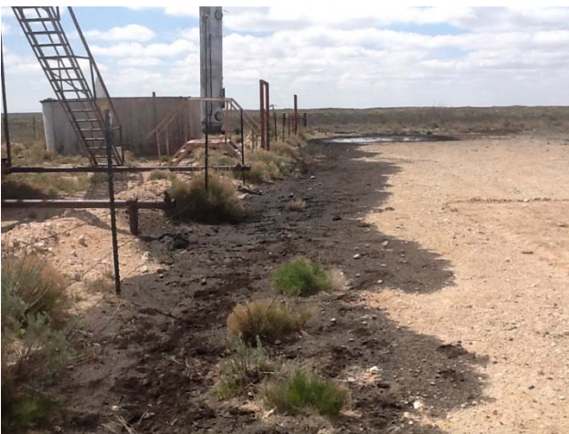
Spill Run North side
