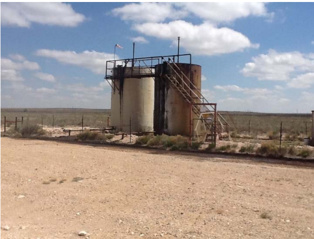
Spill run looking south
