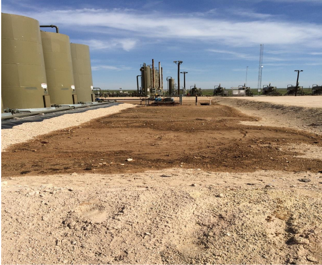
View looking towards the North (3/23/2016)
