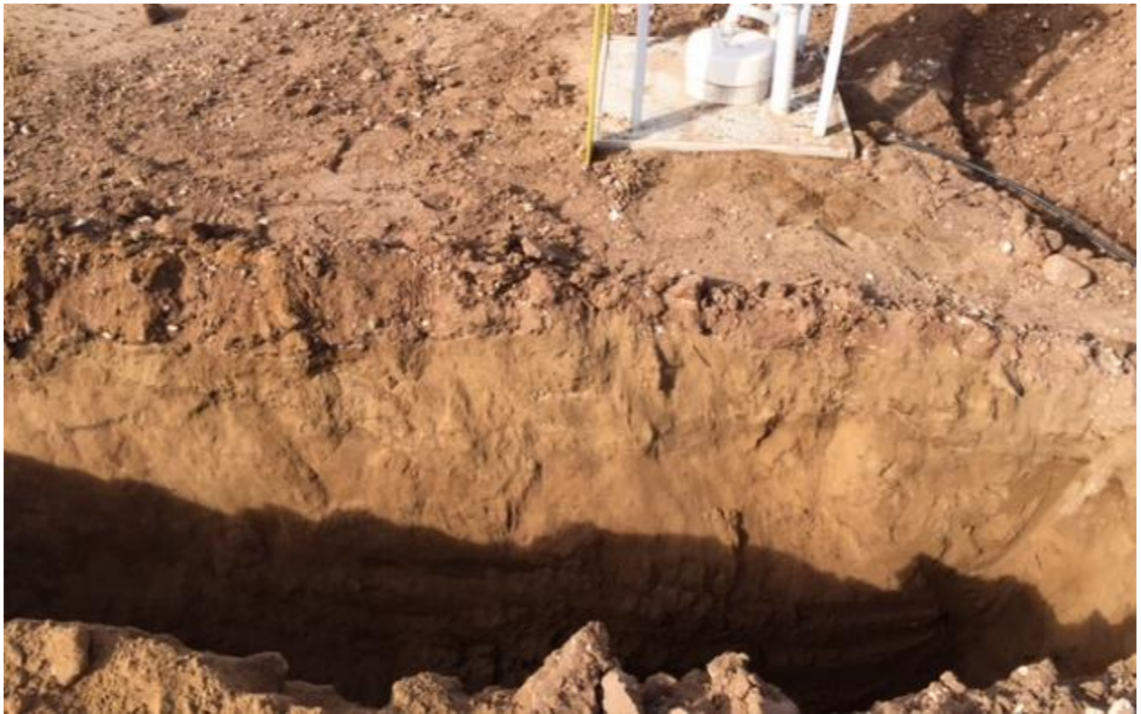
PHOTO 8: View of excavation of affected soil adjacent to cathodic protection system, facing west.
