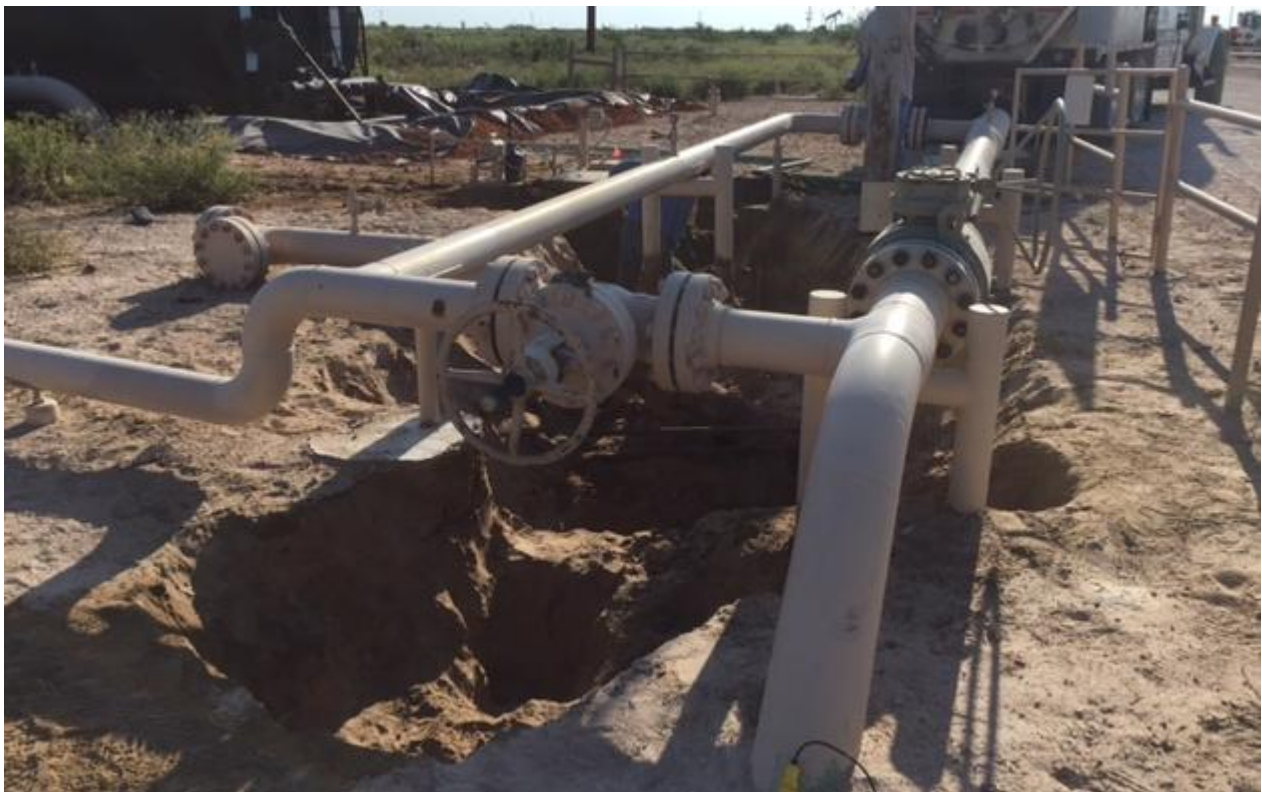
PHOTO 4: View of hydroexcavation activities under facility piping, facing east.
