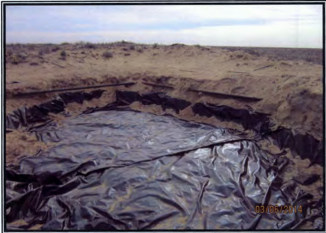
5. View of SP3 following liner installation and seating.
