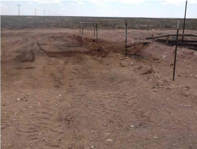
Surface removal at release point
