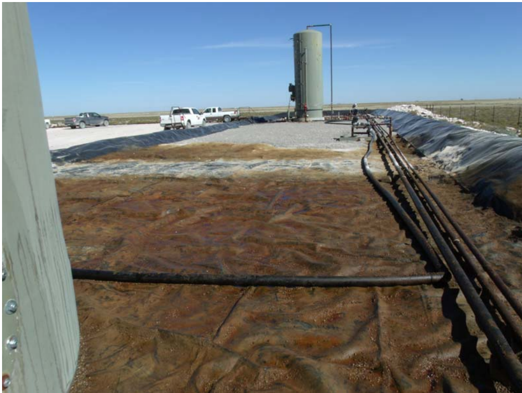
Photograph #5- Release with in containment berm.
