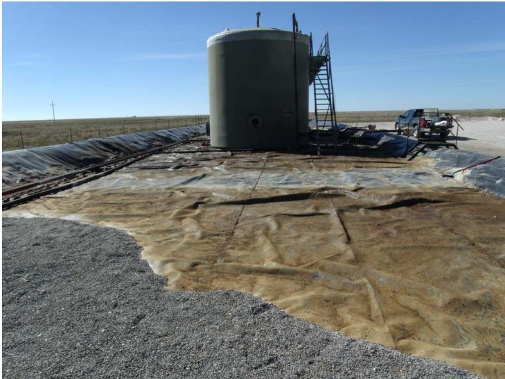
Photograph #6- Release with in containment berm.
