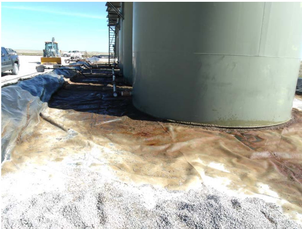
Photograph #1- Release with in containment berm.
