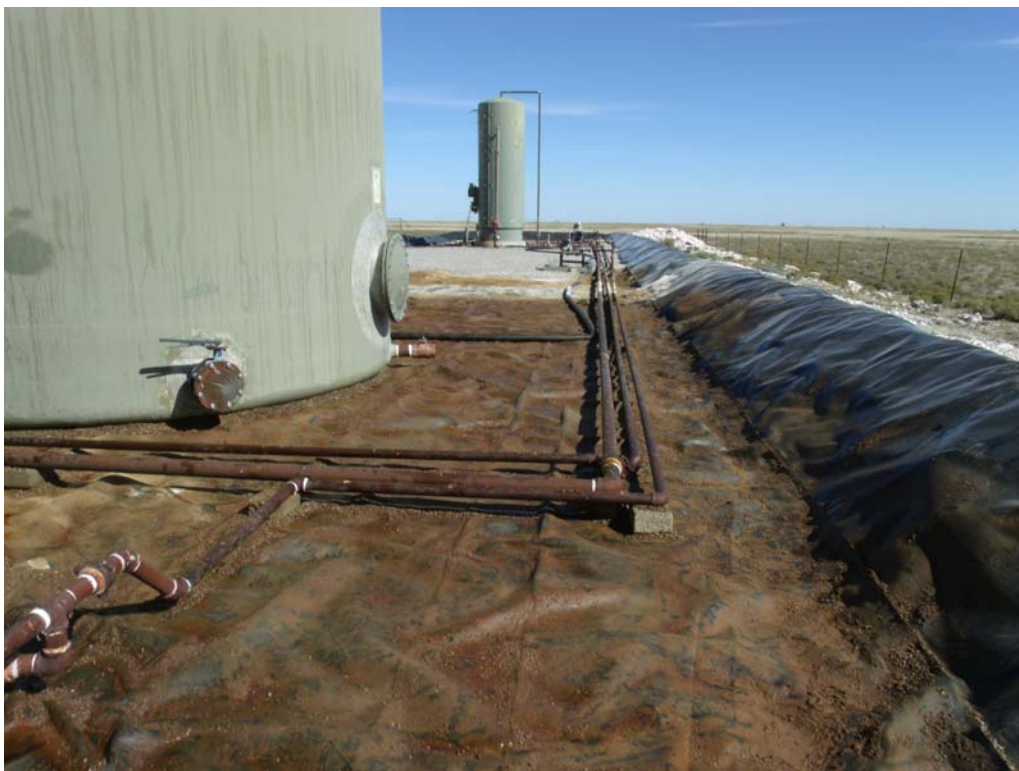
Photograph #4- Release with in containment berm.
