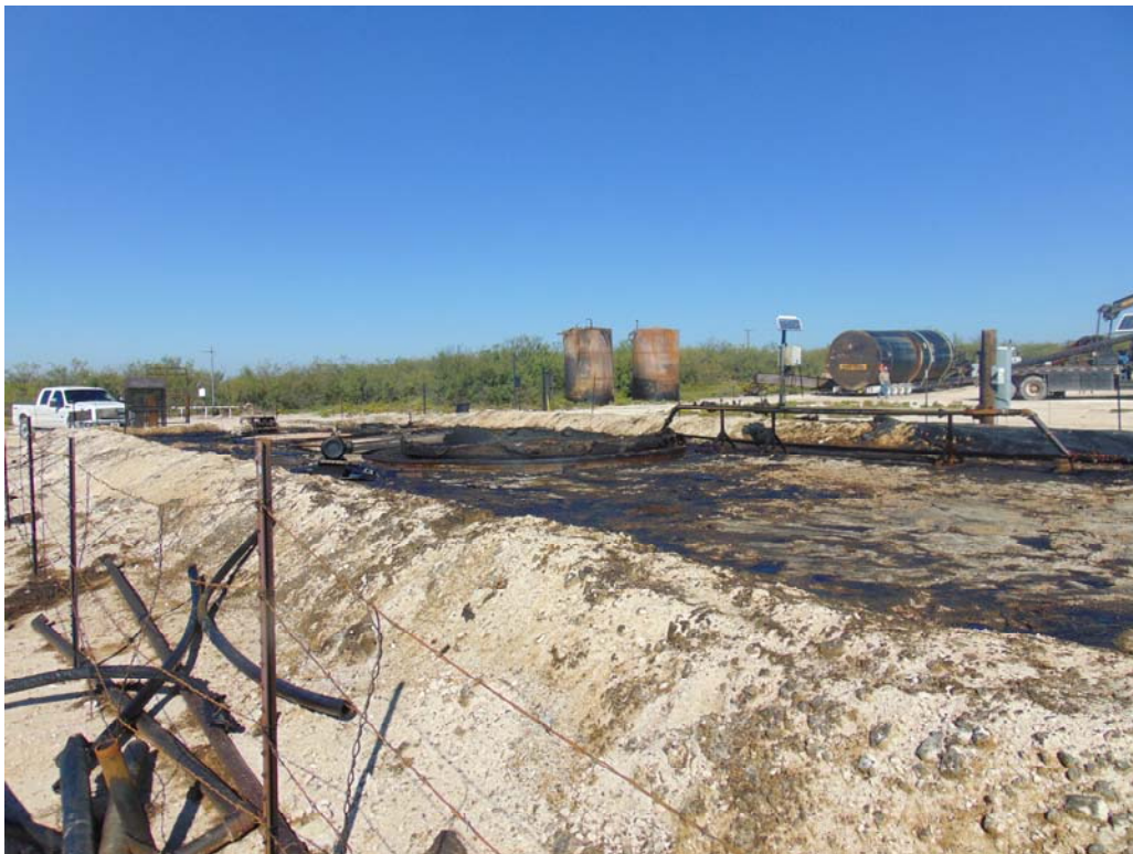
Photograph #2 – Tank battery struck by lightning
