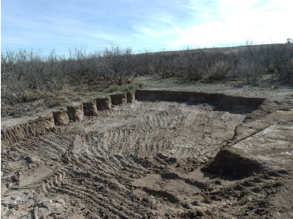
Photograph #5 – Blending the soil around SP4
