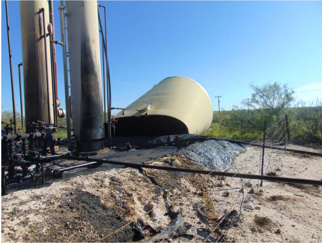
Photograph #3 – Tank battery struck by lightning
