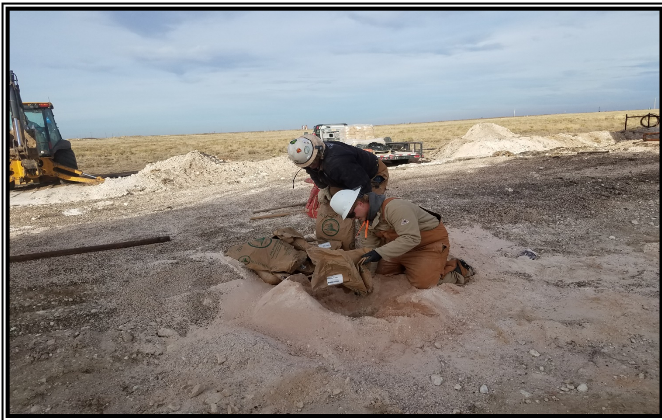
View of emplacement of bentonite plug in boring Middle a during plugging and abandonment.
