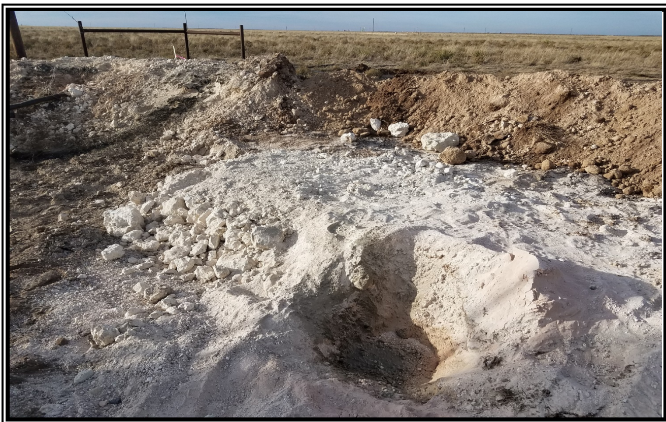
View of boring NW a after plugging and abandonment.
