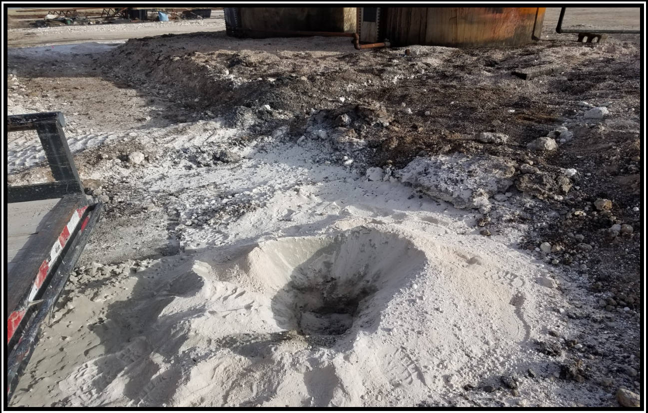
View of of boring N1 after plugging and abandonment.
