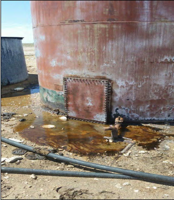
Photograph 3 - A third view looking at the released fluids within tank battery secondary containment.
