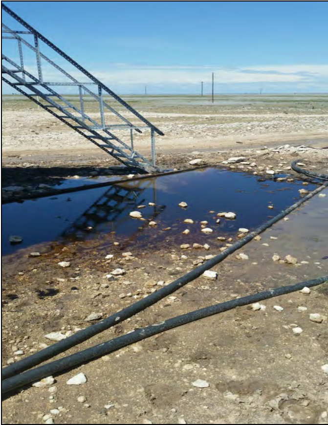
Photograph 1 - A view looking at the released fluids within tank battery secondary containment.
