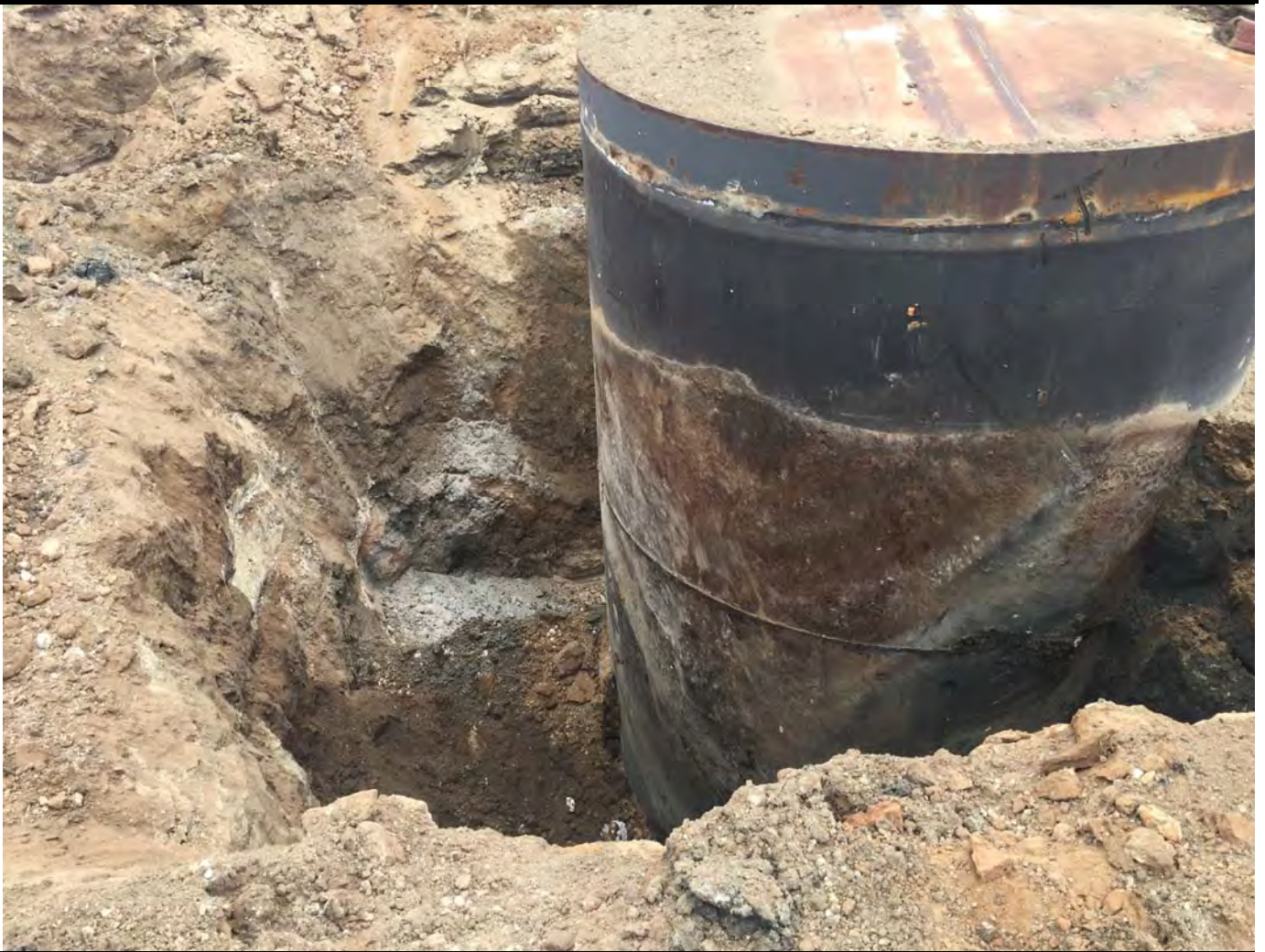
Photo 3: View of preparation to removal the northern field scrubber BGT.
