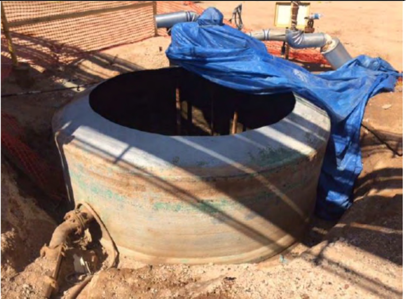
Photo 2: View of the West Boiler Sump after cutting top off, facing southwest.
