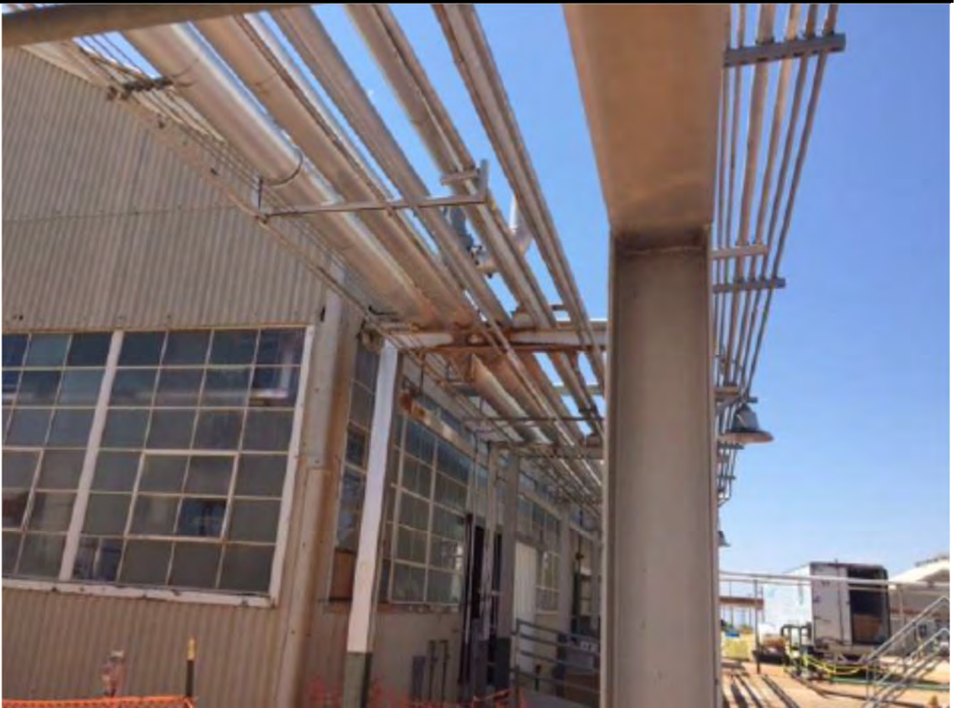
Photo 6: View of affected pipe rack support and associated utilities, included the high pressure steam line, facing south.
