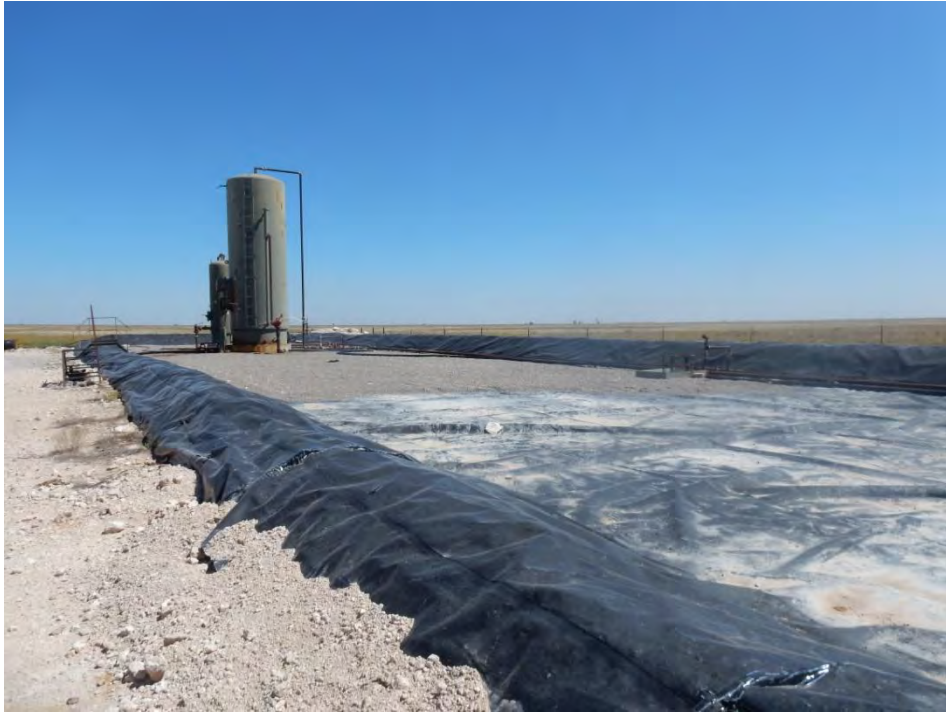
Site Prior to Remediation Showing Split in Liner September 14, 2017
