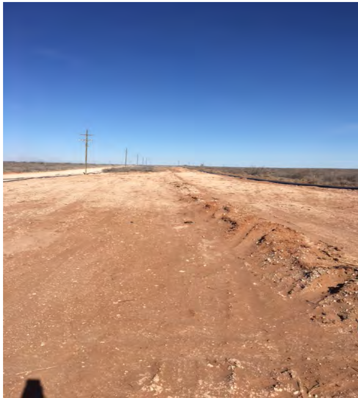
Photo 3 - Backfilled excavation and wheel compacted
