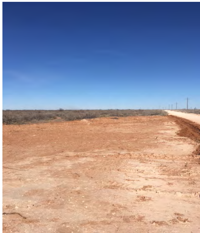
Photo 4 - Backfilled excavation and wheel compacted
