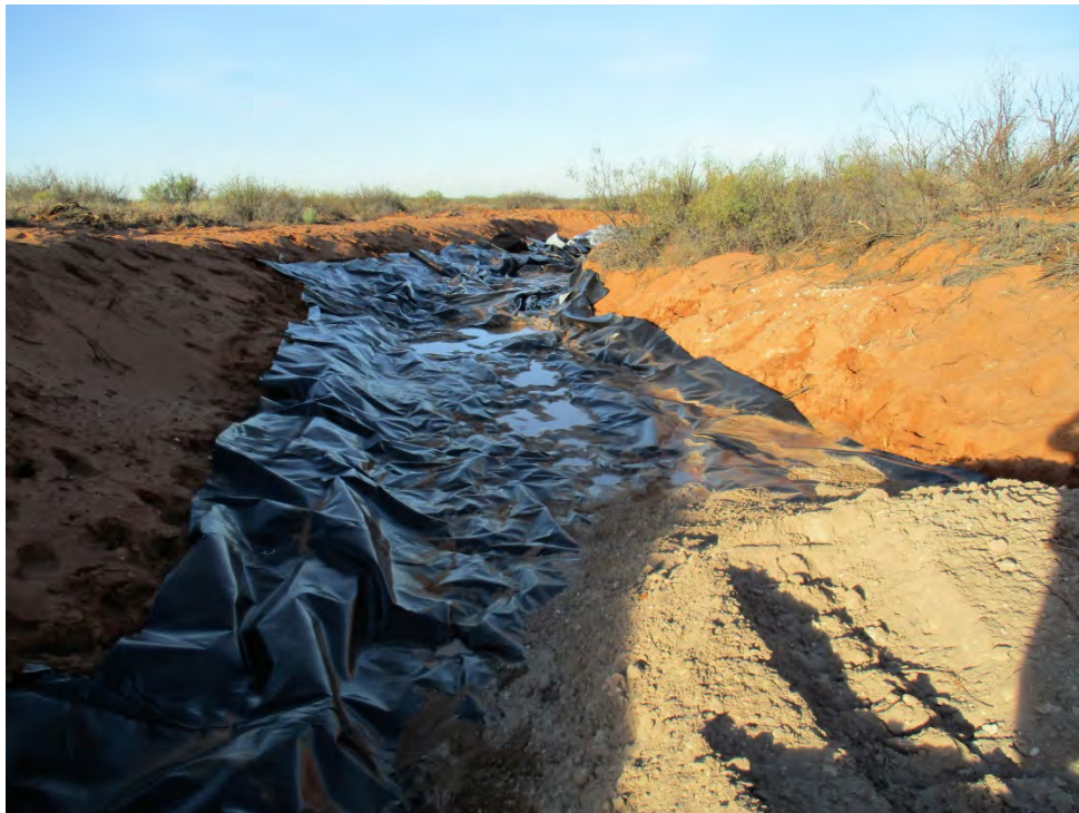
Photo 1 - Liner placement
