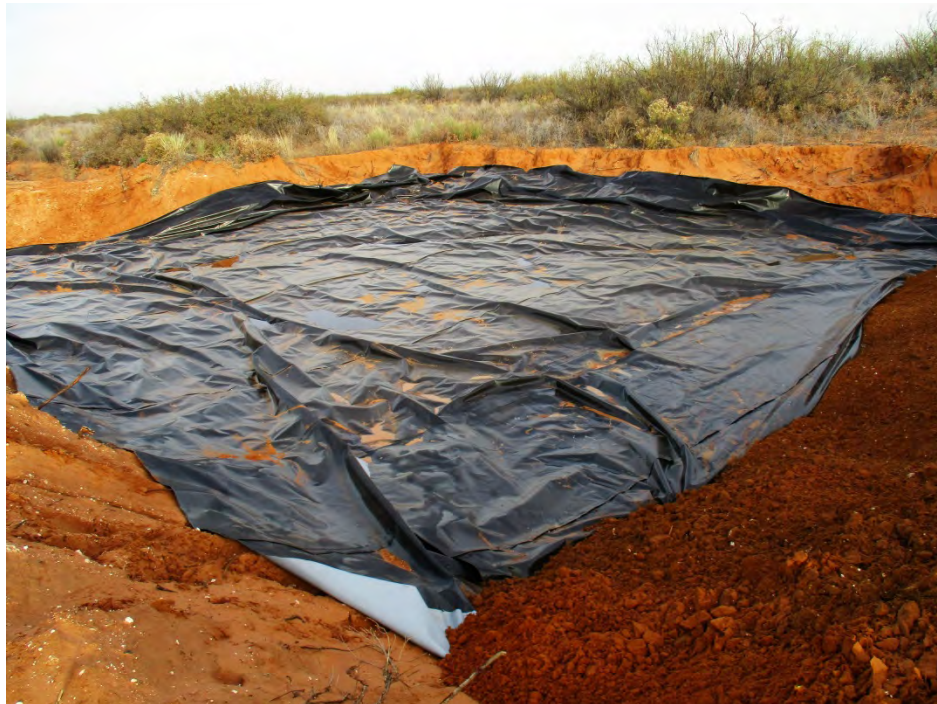
Photo 2 - Liner placement
