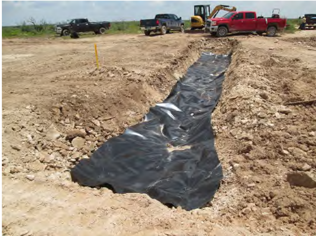
View East – Excavation area with 40 mil liner to the north of the water pipeline.
