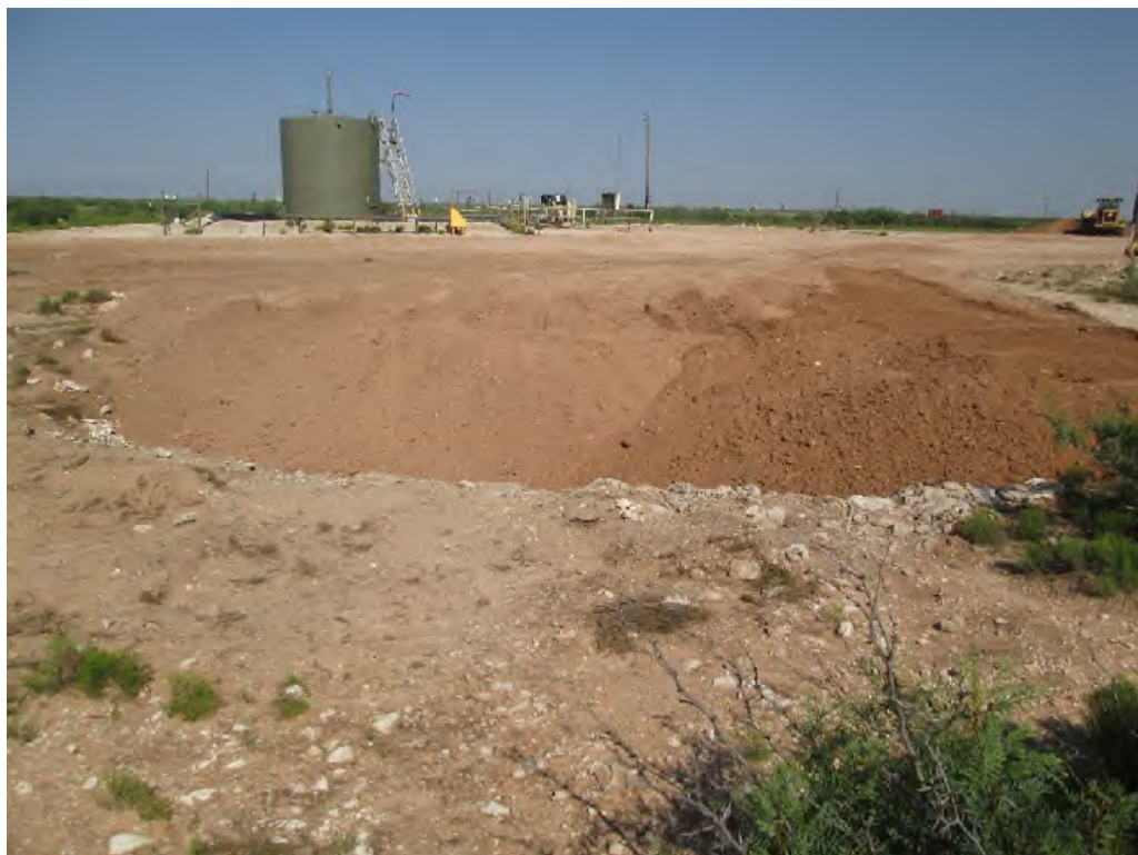
View West – Backfilled excavation prior to final grading.
