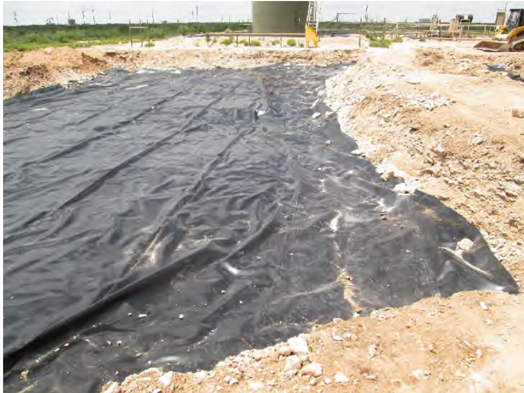
View West – Excavation area with 40 mil liner.
