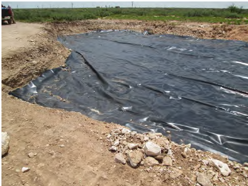
View Southeast – Excavation area with 40 mil liner.
