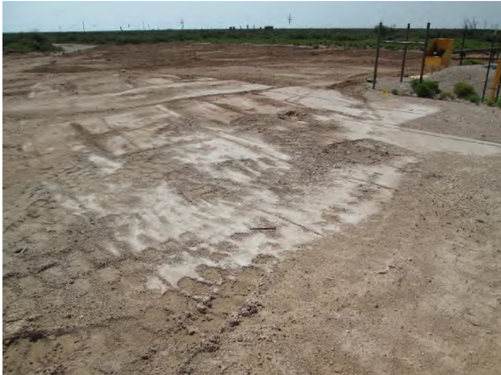
View Southeast – Backfilled excavation with final grading.
