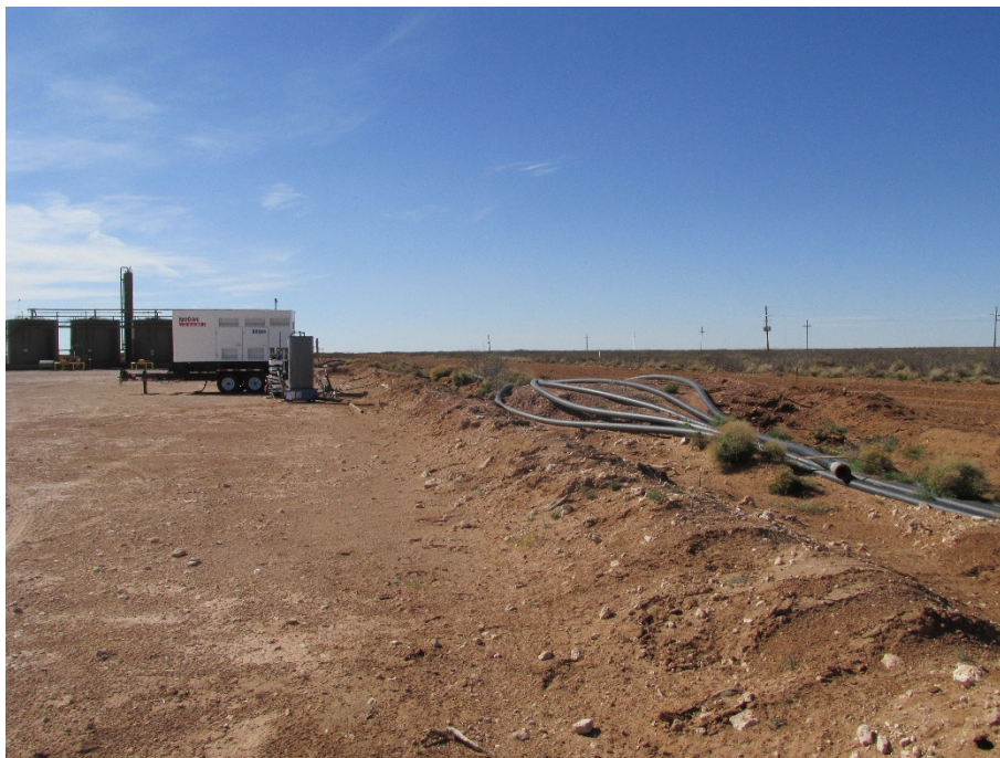
Photo 4 - Backfilled excavation and wheel compacted
