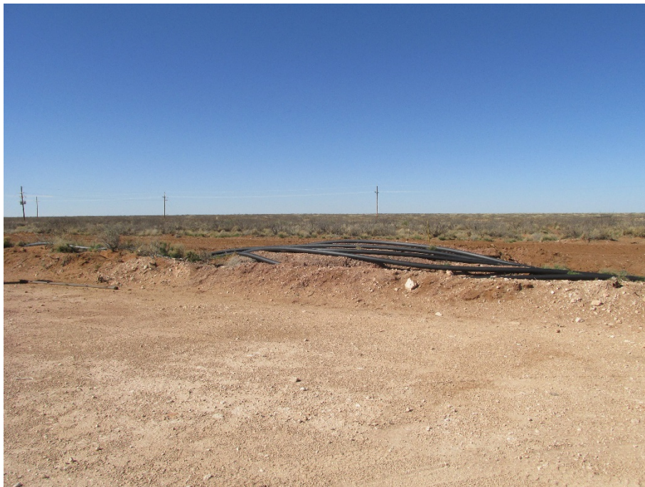
Photo 4 - Backfilled excavation and wheel compacted
