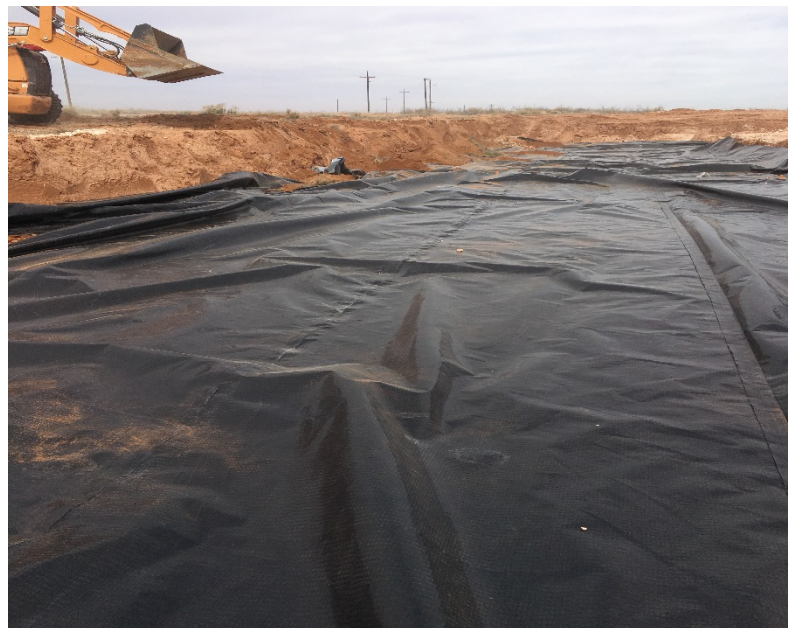
Photo 2 - Liner placement
