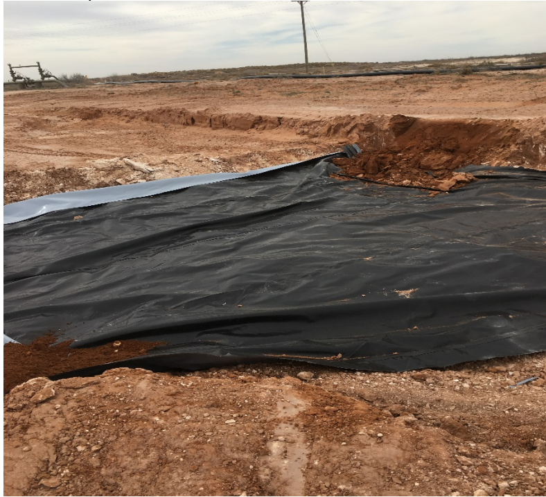
Photo 1 - Liner placement
