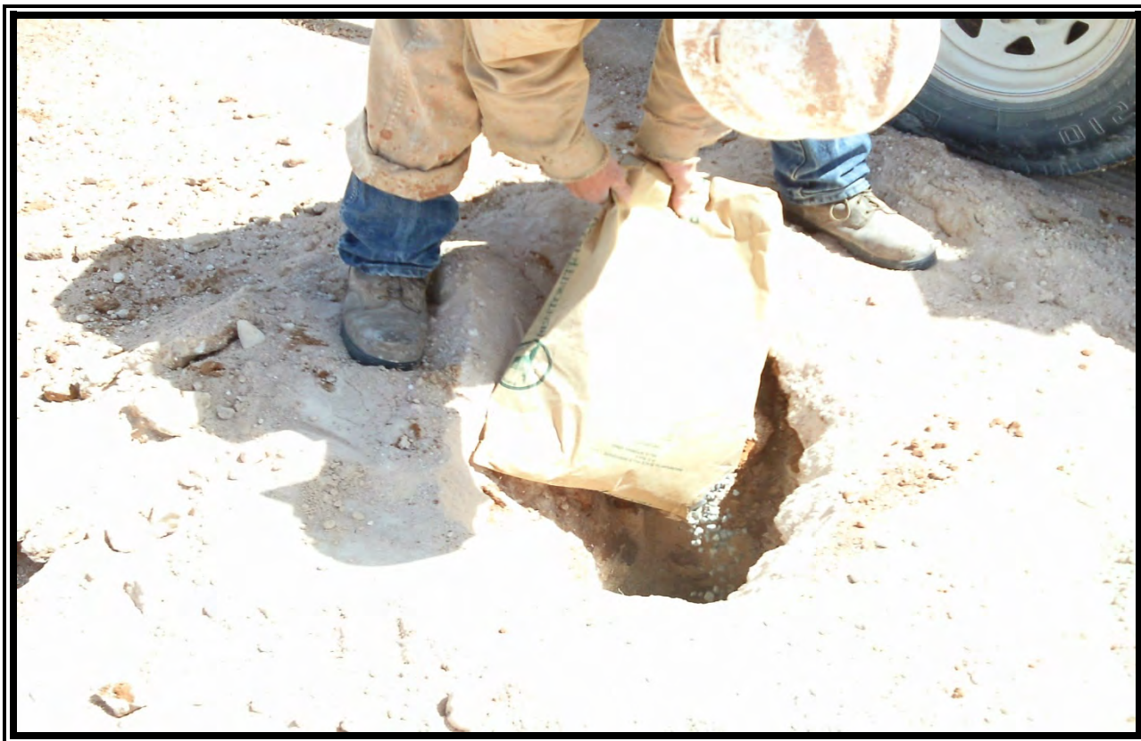
View of emplacing bentonite pellets in soil boring.
