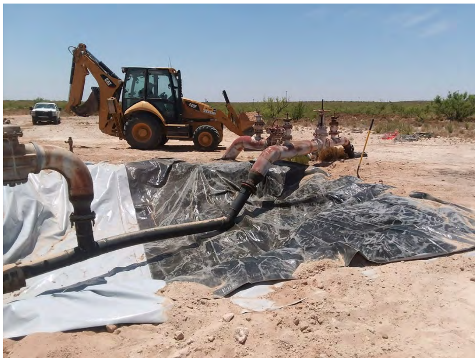
Photo 2 - Placement of liner
