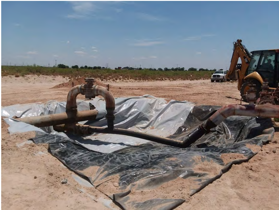
Photo 1 - Placement of liner
