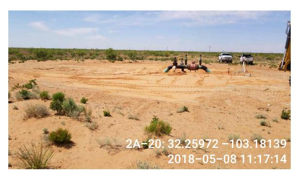
Photo 2 - Backfilled excavation
