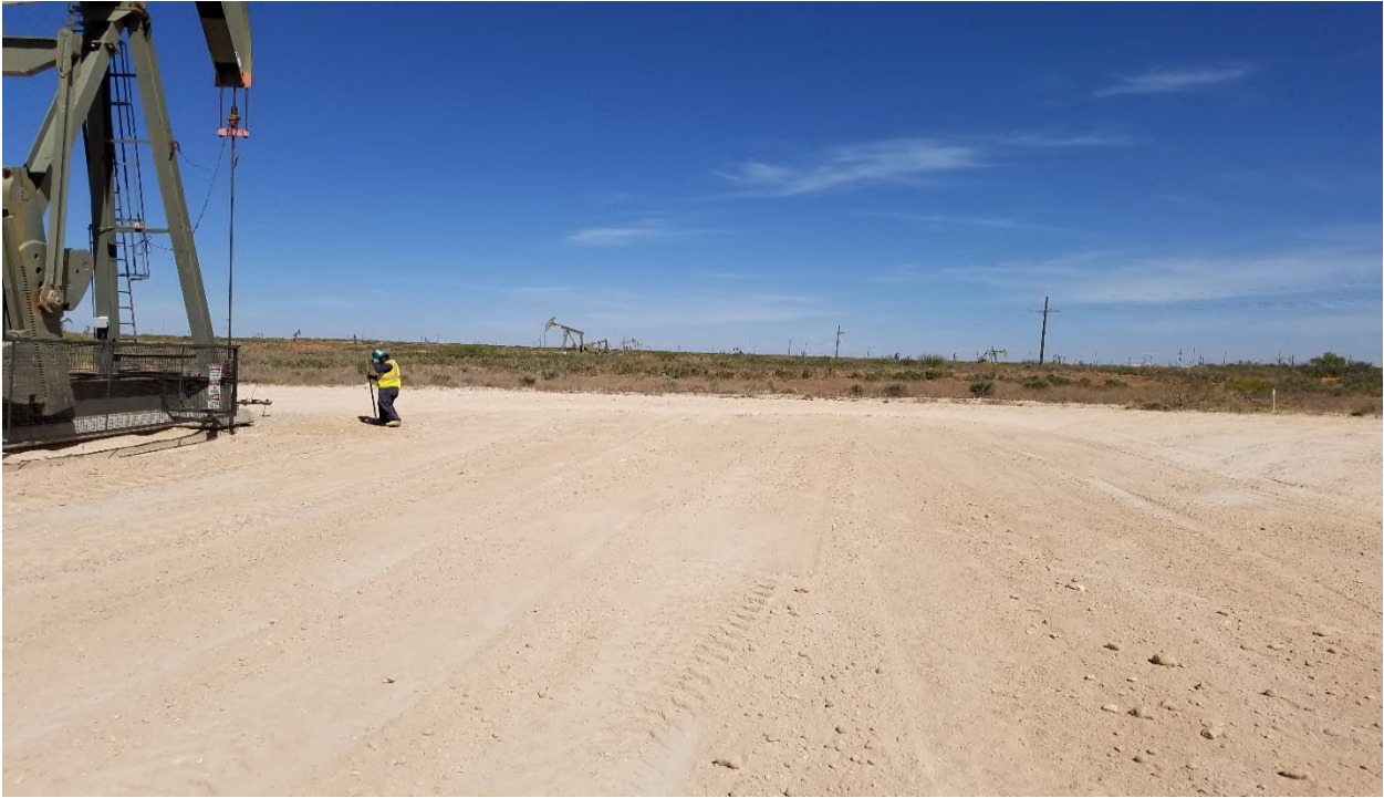
Photo 9: Eastern view on southern side of pumping unit after backfilling with imported caliche (04/18/2018).
