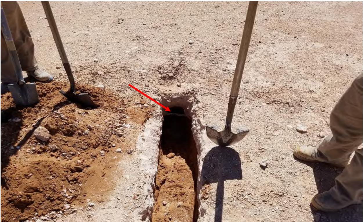
Photo 6: closeup view of exposed 440-volt power line from southwest corner of pad to panel at pumping unit [power line denoted by “red” arrow] (04/17/2018).
