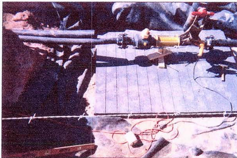
Floor Construction of New Plastic Box with Poly Liner (130 ft East)
