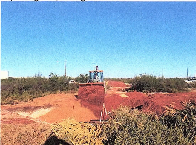
Backfilling above the liner, facing southeast
