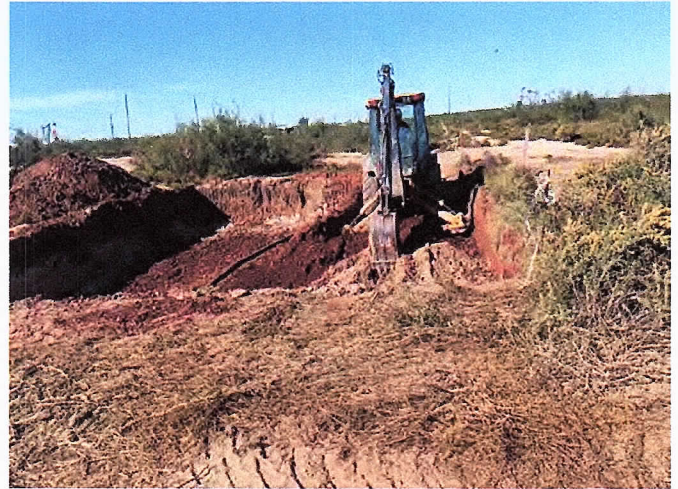
Excavating the site to 5 ft bgs, facing north
