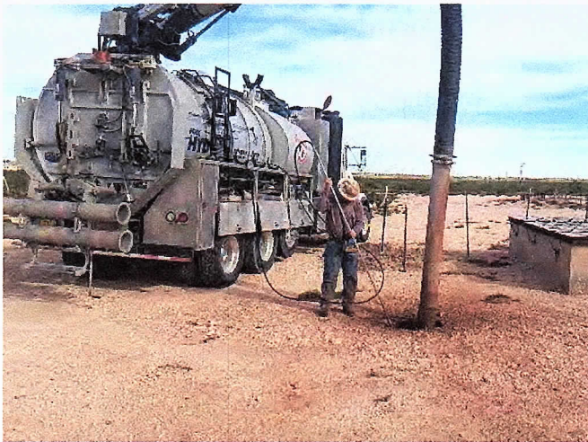
Spotting lines with hydrovac, facing east
