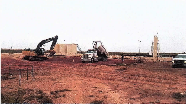
Backfilling the excavation with imported soil, facing southwest 12/6/2017
