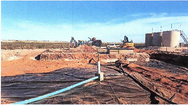
Padding the 20-mil, reinforced liner with imported blow sand, facing east 11/29/2017
