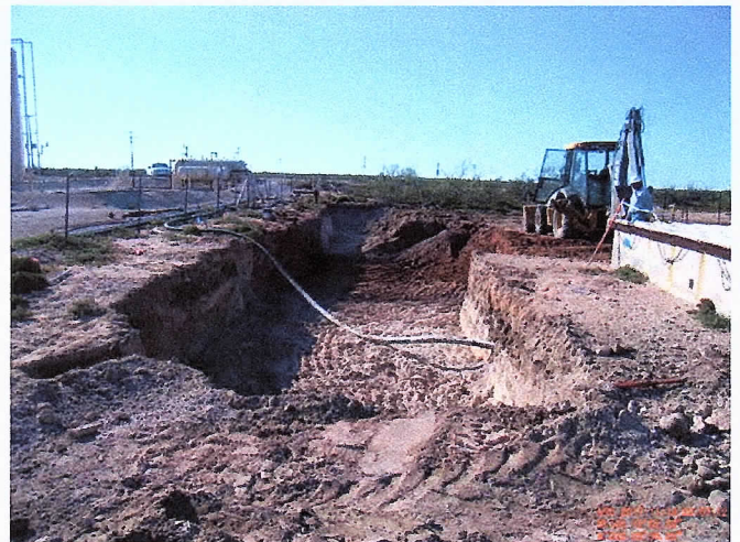
Excavating the site to 5 ft bgs, facing west
