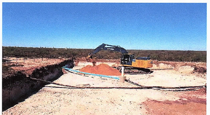
Padding excavation with imported blow sand, facing north
