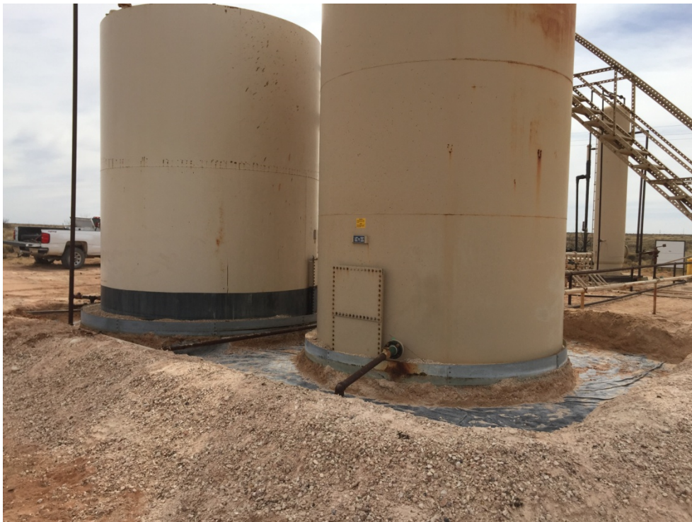
Produced Water Tank and Spill Origin Following Removal of Gravel March 9, 2018
