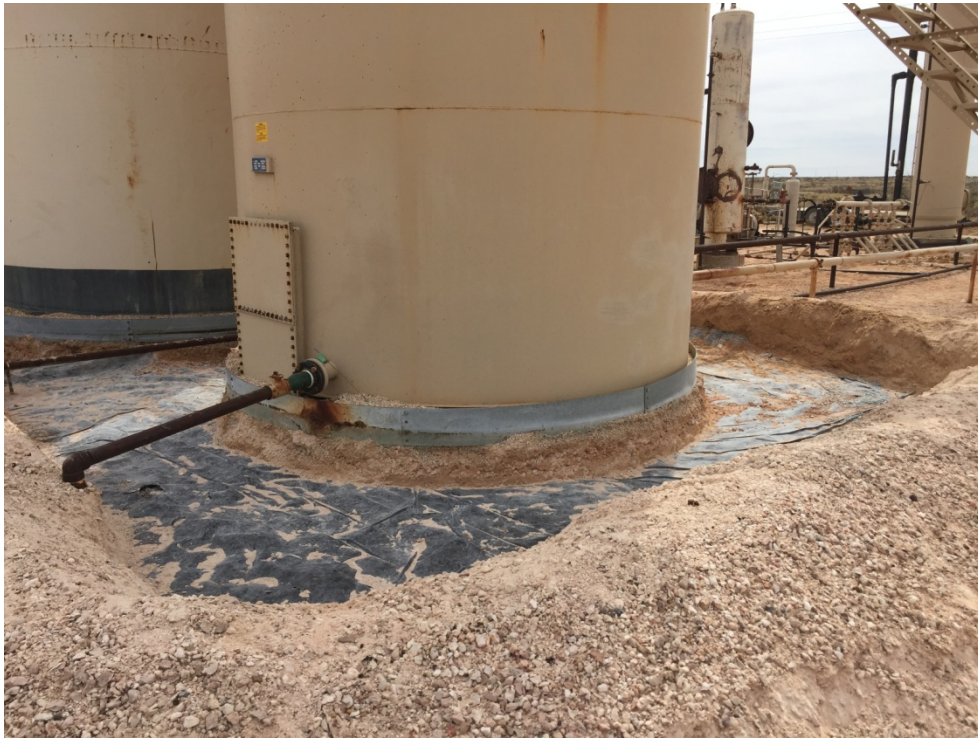
Poly Liner beneath Produced Water Tank Following Removal of Gravel March 9, 2018
