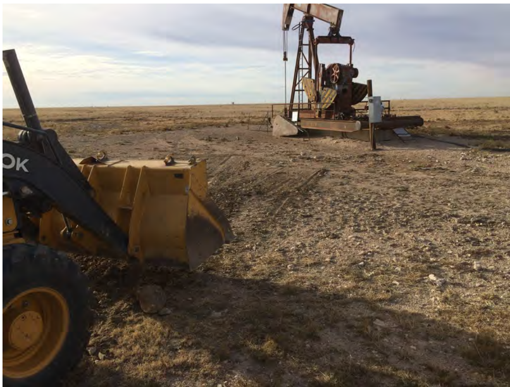
Exhibit C: Backfilling trench sample at SE Pad. Hard caliche encountered at 1-foot below ground surface. Total depth was 2-feet below ground surface.
